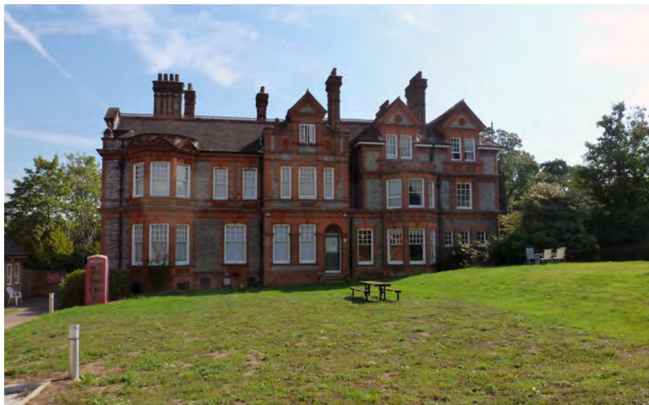
Fig.3: Existing poor quality amenity space serving the occupants of Hillside House
