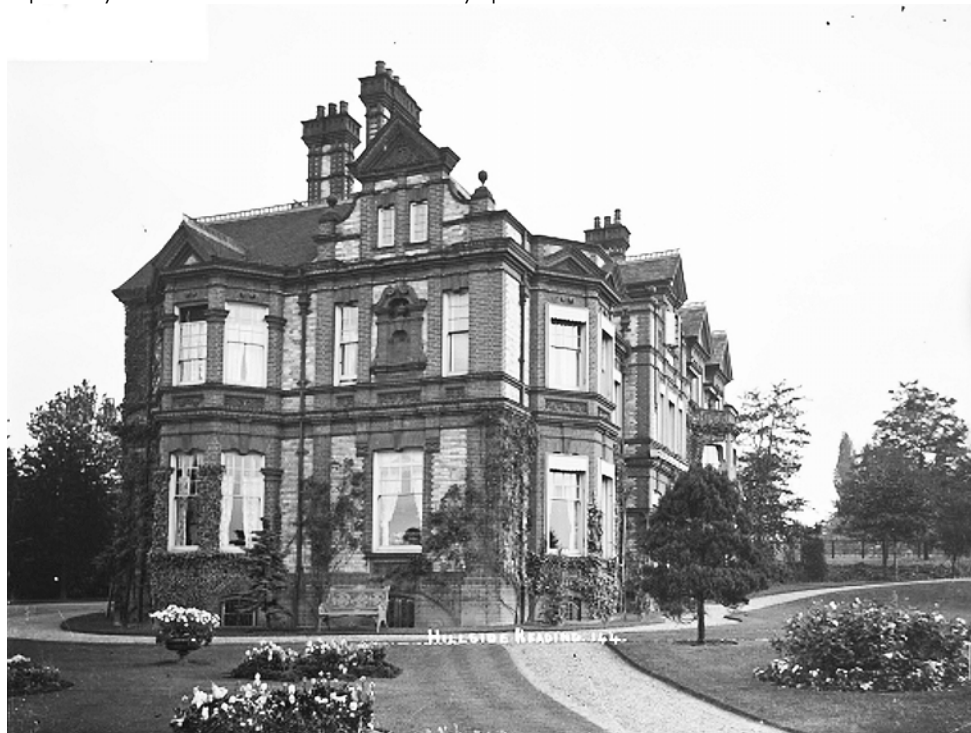
Fig.7: Historic photograph of Hillside House and garden. Image courtesy of the Museum of English Rural Life
