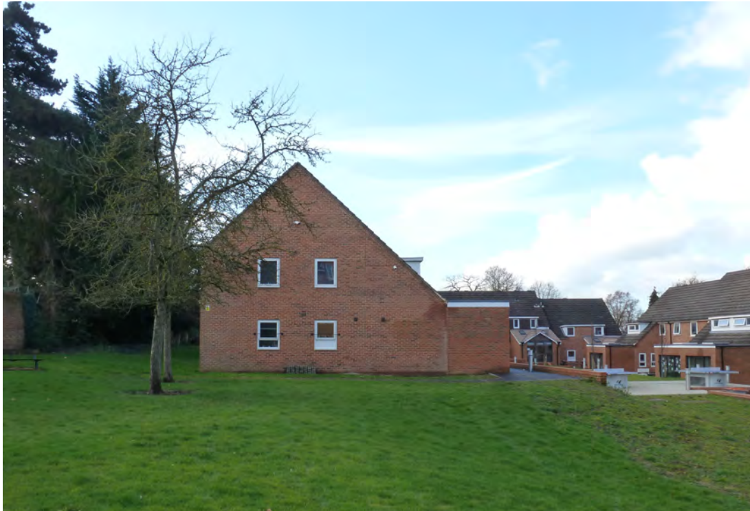
Fig.14: Photograph of east elevation of Hillside Court Block D which faces Hillside House.
