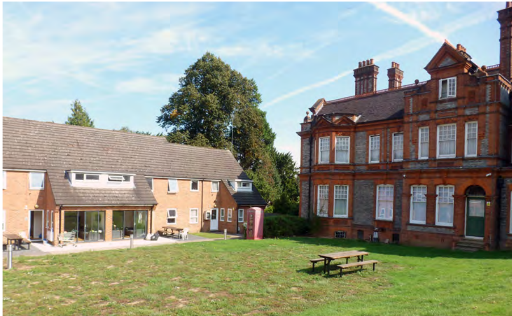
Fig.6: Photograph illustrating Block A's detrimental effect on the setting of Hillside House, there is also no privacy between the external amenity spaces associated with different uses.
