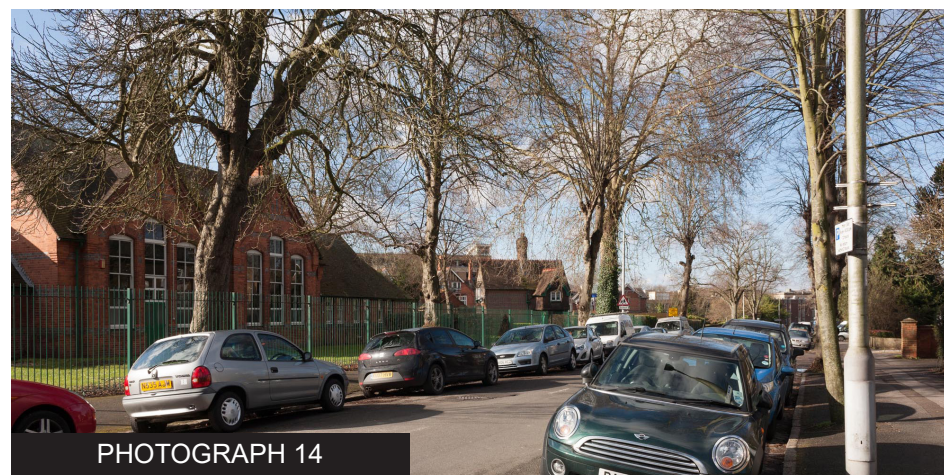
PHOTOGRAPH 14 School Buildings fronting Erleigh Road, looking north
