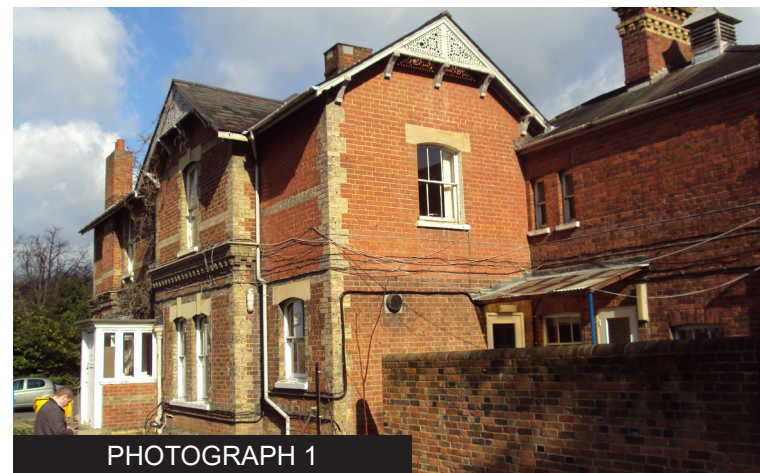
Number 3 Craven Road viewed from the front garden to the south
