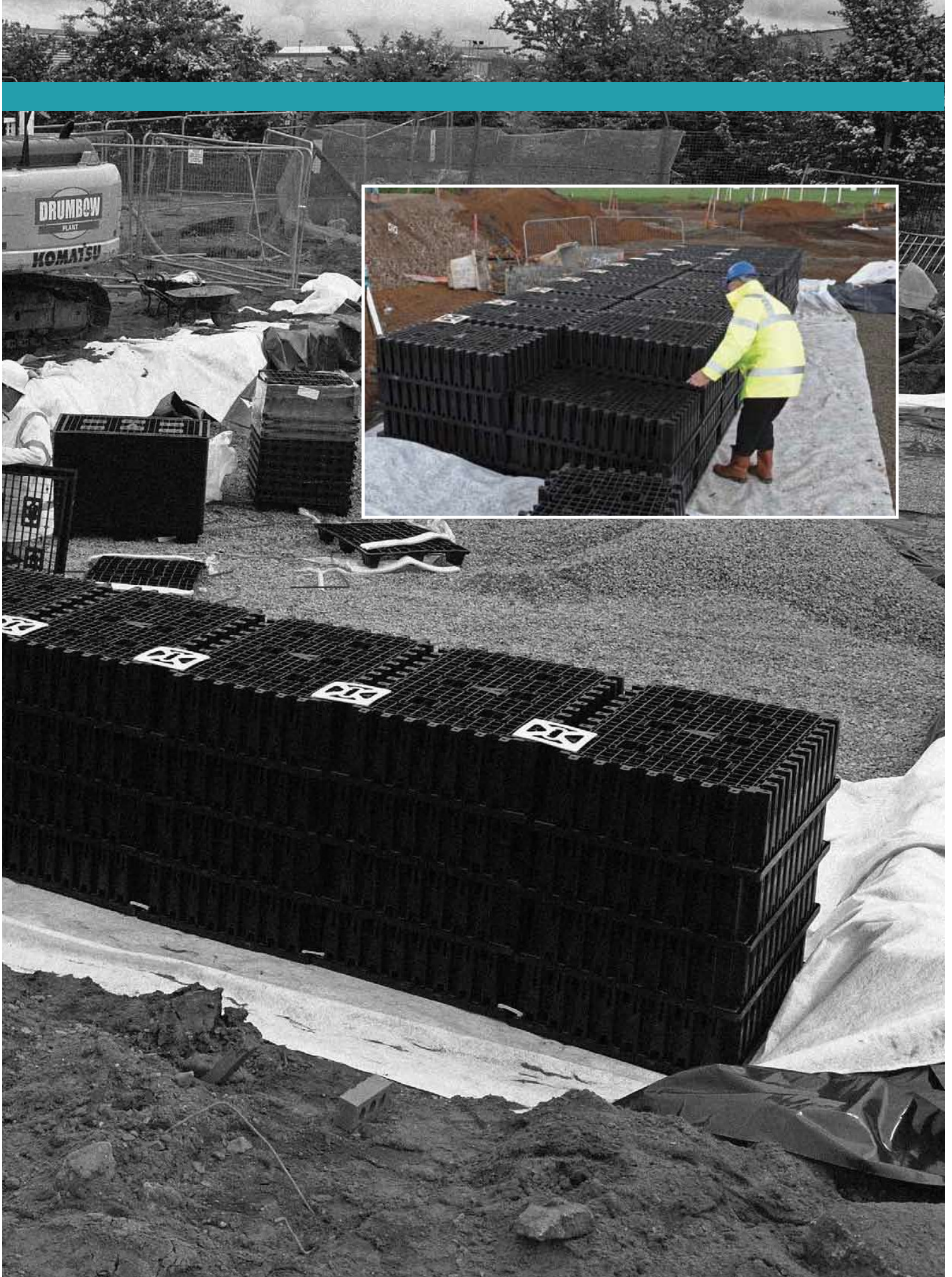
Attenuation tank for Robertson Homes, Seaforth Road, Ayr
