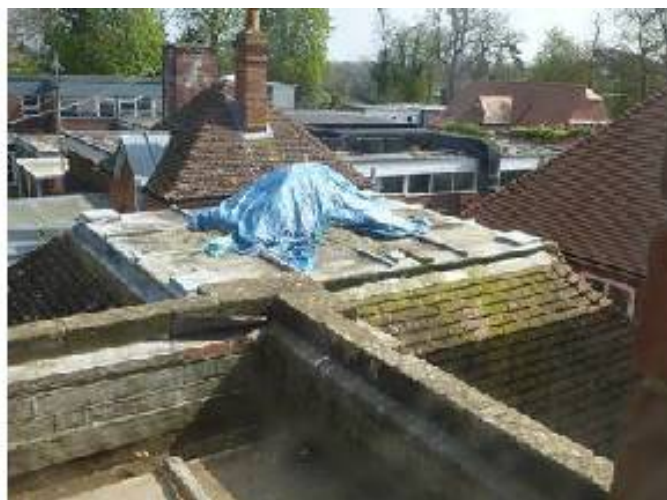
"T" CLASSROOM FLAT ROOF
