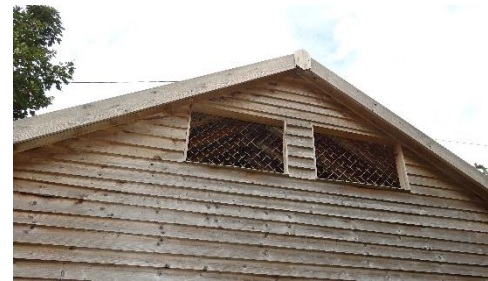
B1: Rear view of building
