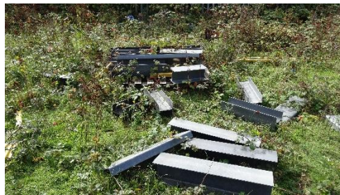
TN13: Construction materials
