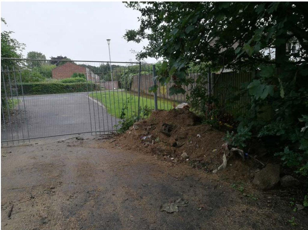
Plate 16 – Site access looking east towards Cadogan Close and the main road
