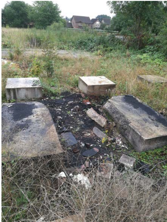
Plate 10 – View of concrete bases and evidence of fires on central western portion of site
