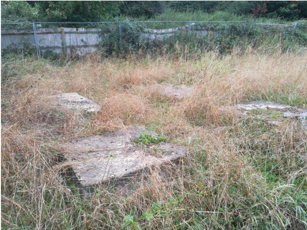
Plate 9 – View of concrete bases within the north eastern corner of the site looking east
