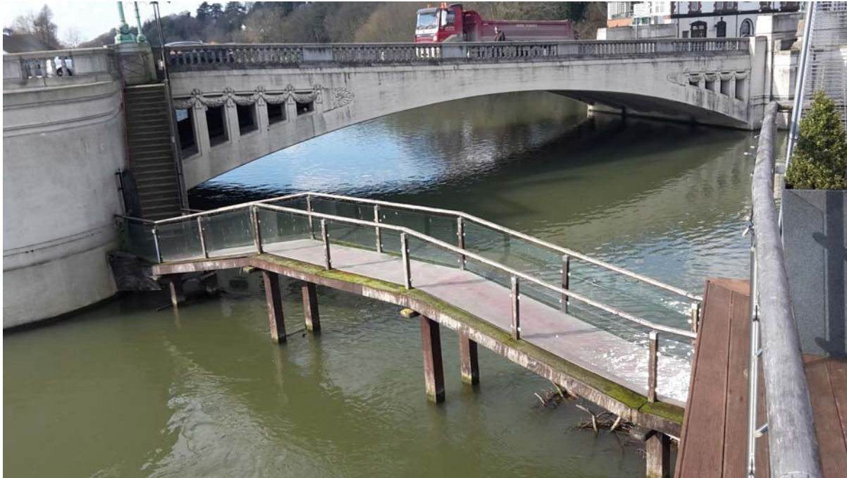
Fig 4. Image of current wooden bridge, to be replaced with new (metal) bridge
