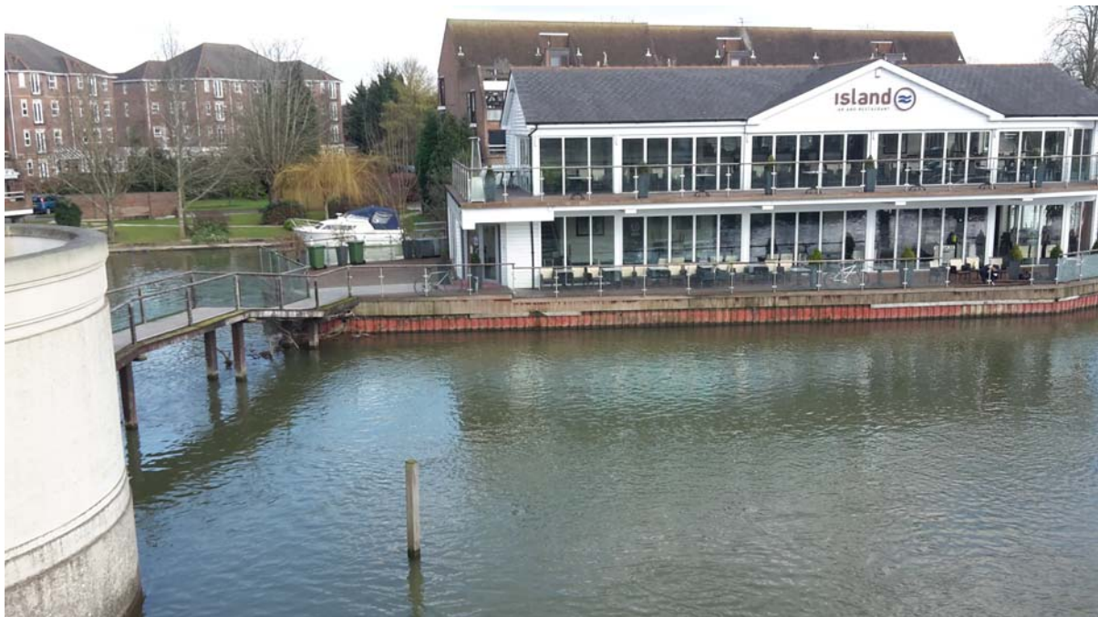
Fig 3. Photo of the Island bar with access bridge in the foreground
