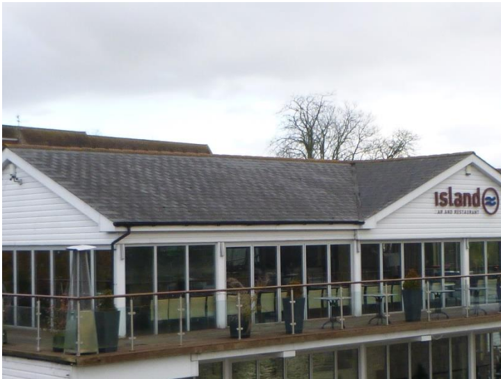
Plate 4. The roof is finished with flat, interlocking tiles.
