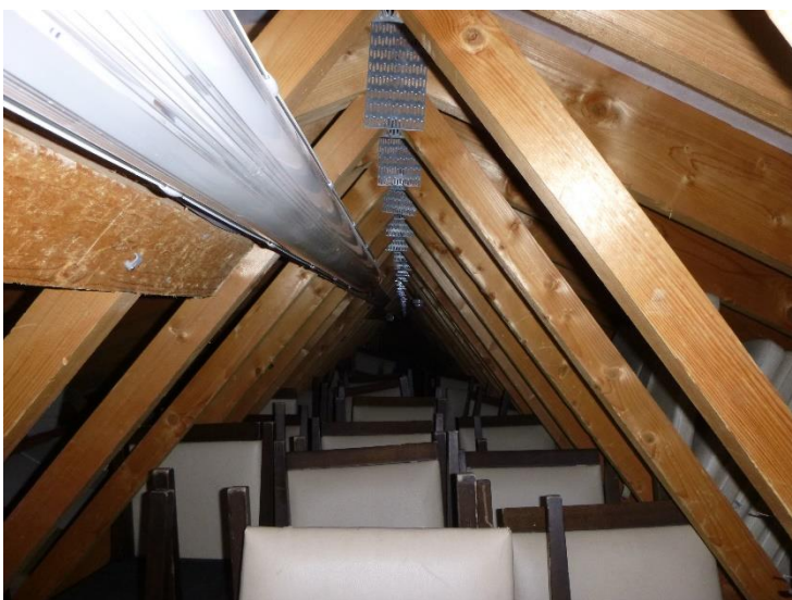
Plate 6. General view of the internal void space.
