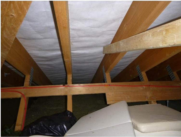
Plate 7. The roof lining is in sound condition.
