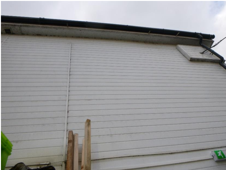
Plate 5. The plastic boarding that forms the walls is in sound condition.
