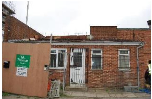
Photograph 4. The single-storey sloping roof extension to the north-western corner of Building 2.
