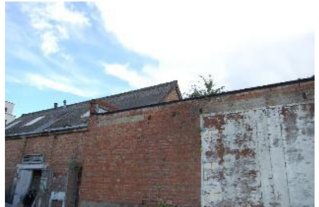
Photograph 22. The western elevation of Building 5.
