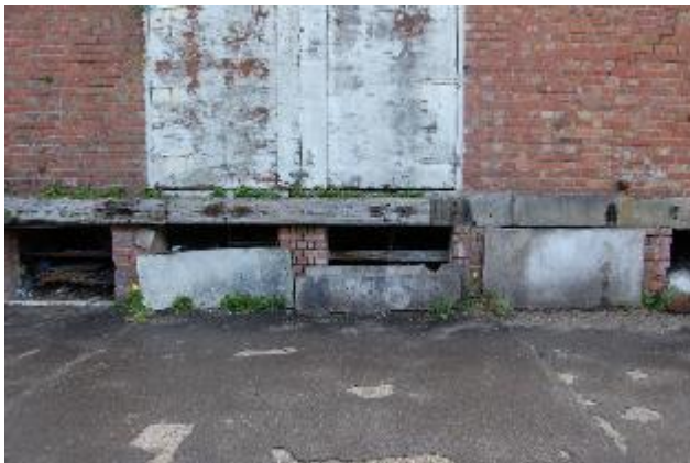
Photograph 23. Showing the raised height of Building 5.
