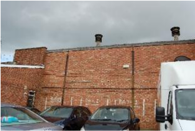
Photograph 7. The western elevation of Building 2.
