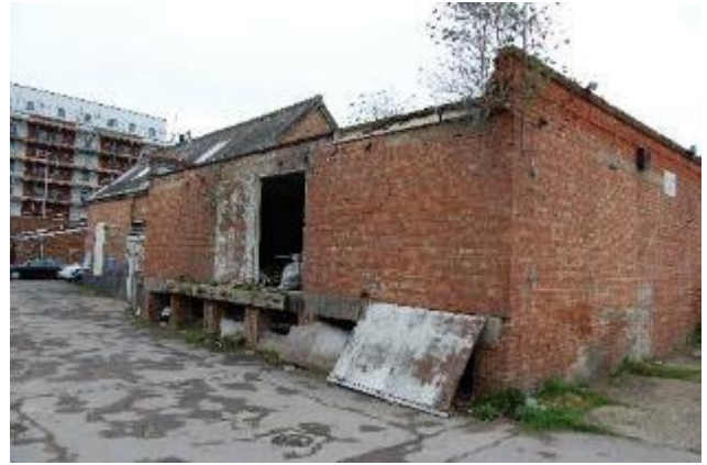
Photograph 8. The western elevation of Building 5.
