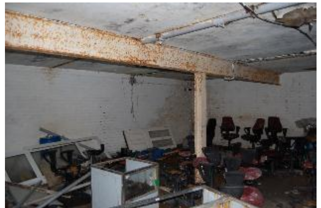
Photograph 24. The interior of Building 5.
