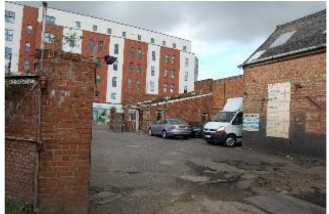
Photograph 26. Showing the tarmacked hard-standing that surrounds the buildings.
