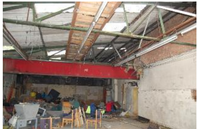
Photograph 10. The interior of Building 2, looking south.
