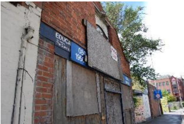
Photograph 15. The northern elevation of Building 3.
