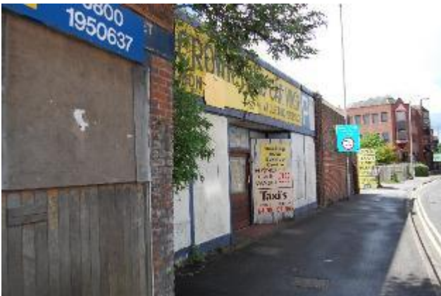
Photograph 9. The northern flat roofed extension of Building 2.
