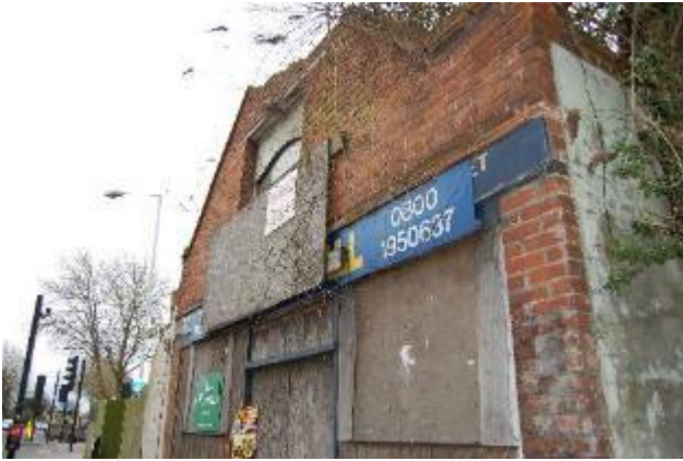
Photograph 7. The northern elevation of Building 3.
