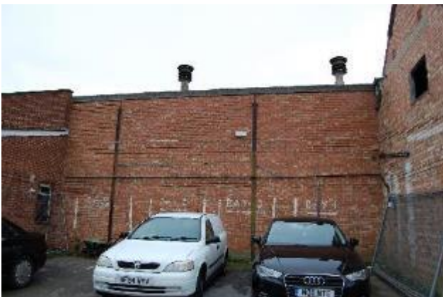
Photograph 3. The western elevation of Building 2.
