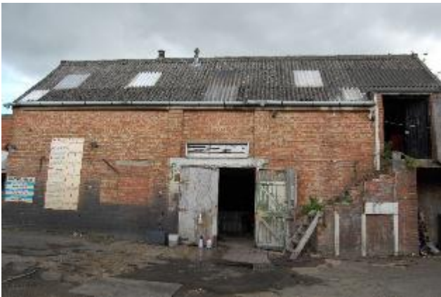
Photograph 1. Building 1 viewed from the west, showing the door to the upper room (far right of the photograph).
