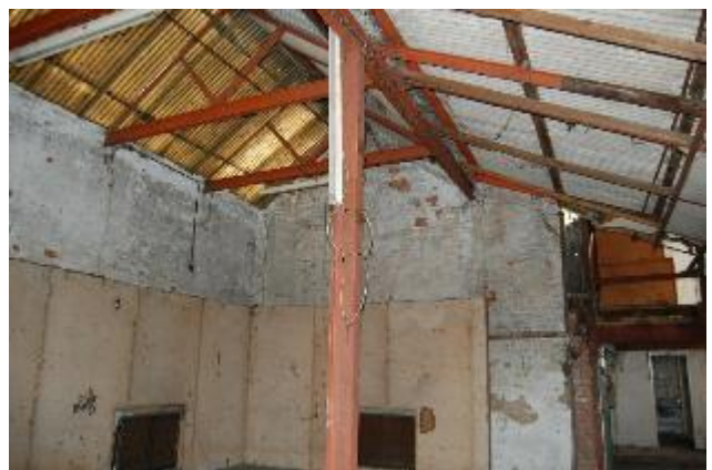
Photograph 18. The second of the large rooms within Building 3 (southern end).
