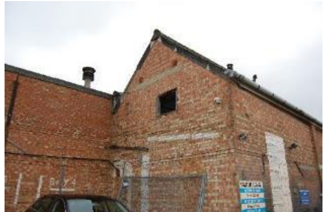
Photograph 2. The northern gable end of Building 1, with barge board features to the apex of the roof.
