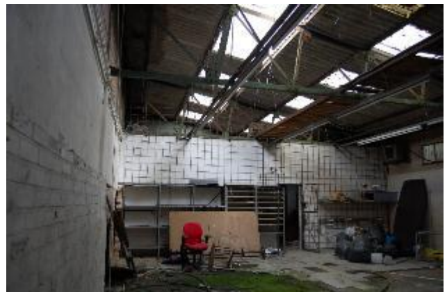
Photograph 12. The flat roofed extension to the north of Building 2 extends into the interior to create a number of rooms.
