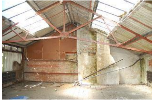
Photograph 20. The upper level of Building 4.
