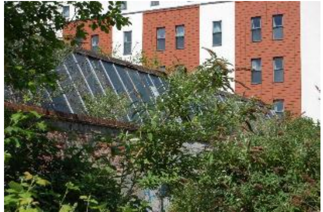
Photograph 14. The eastern elevation of Building 3, showing the glass panelled roof.
