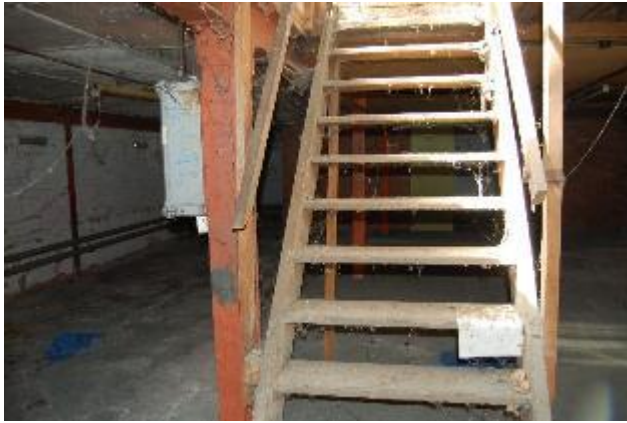
Photograph 19. The ground floor level of Building 4.
