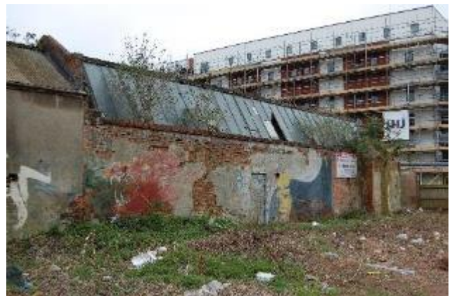
Photograph 6. The eastern elevation of Building 3, showing the glass panelled roof.
