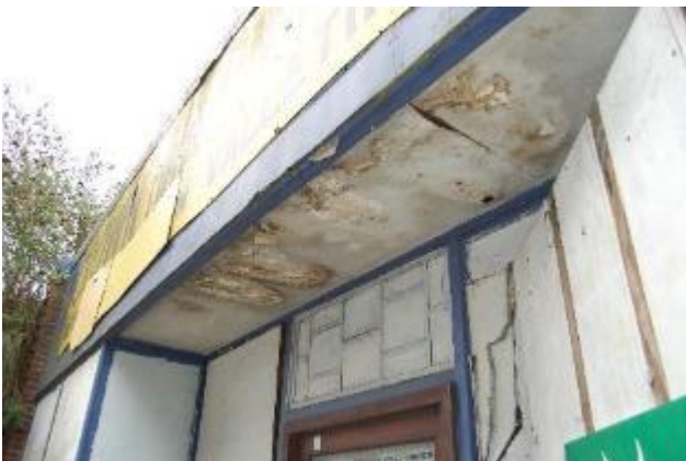
Photograph 5. The northern flat roofed extension of Building 2.
