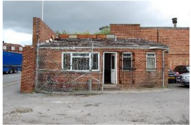
Photograph 8. The single-storey sloping roof extension to the north-western corner of Building 2.
