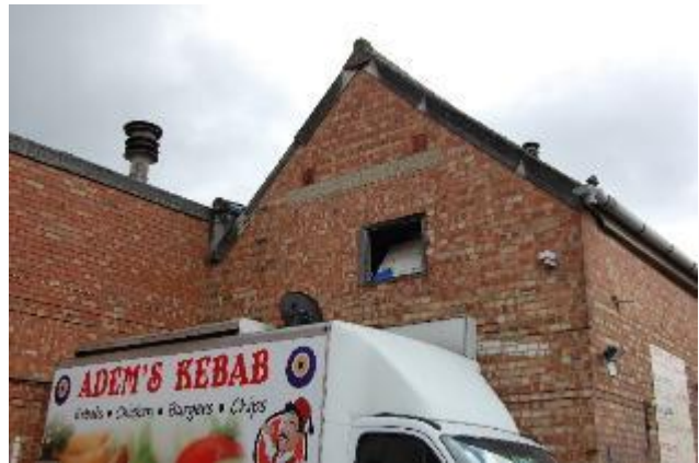
Photograph 2. The northern gable end of Building 1, with barge board features to the apex of the roof.
