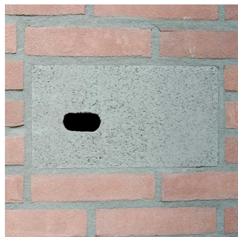
Figure 3. Example of a Woodstone Build-in Swift Box integrated into a wall
