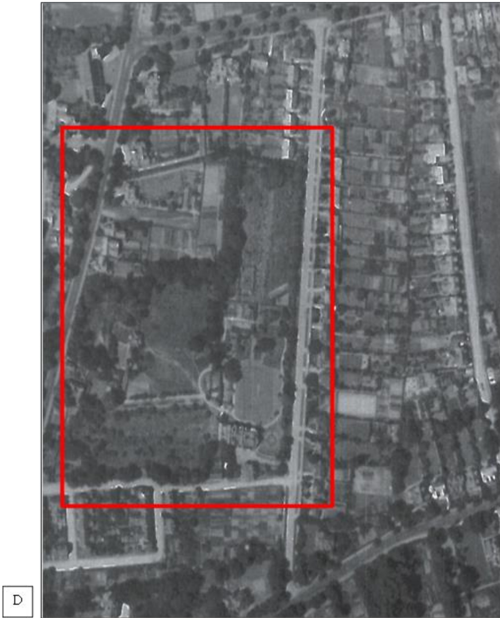
Figure 7 Aerial Photo taken by the RAF, 4237 1646, 10-7-46, 541 Squadron. Image Courtesy of the National Monument Record (licence)
