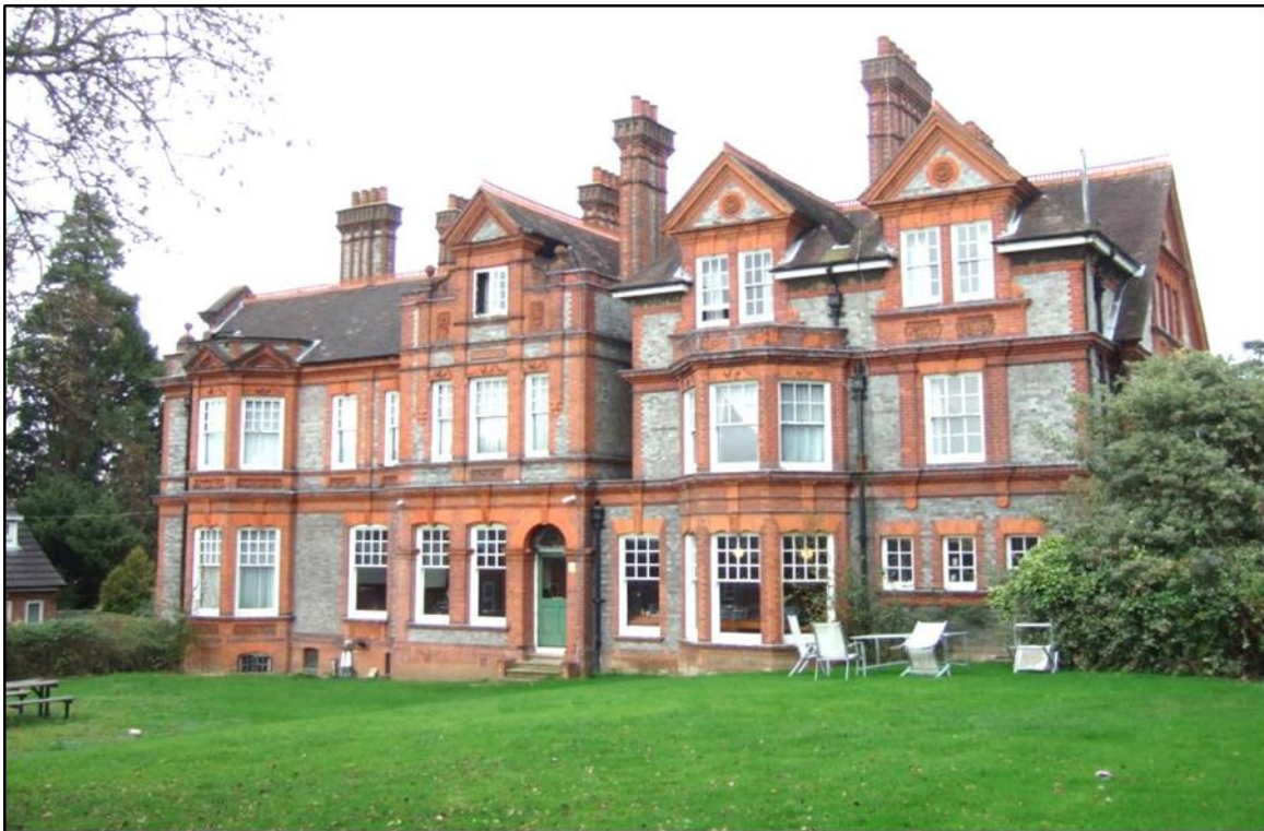
Figure 14 West elevation of Hillside showing sloping lawn, proximity of University block and overgrown holly on the south west corner. Gaila Adair 2016
