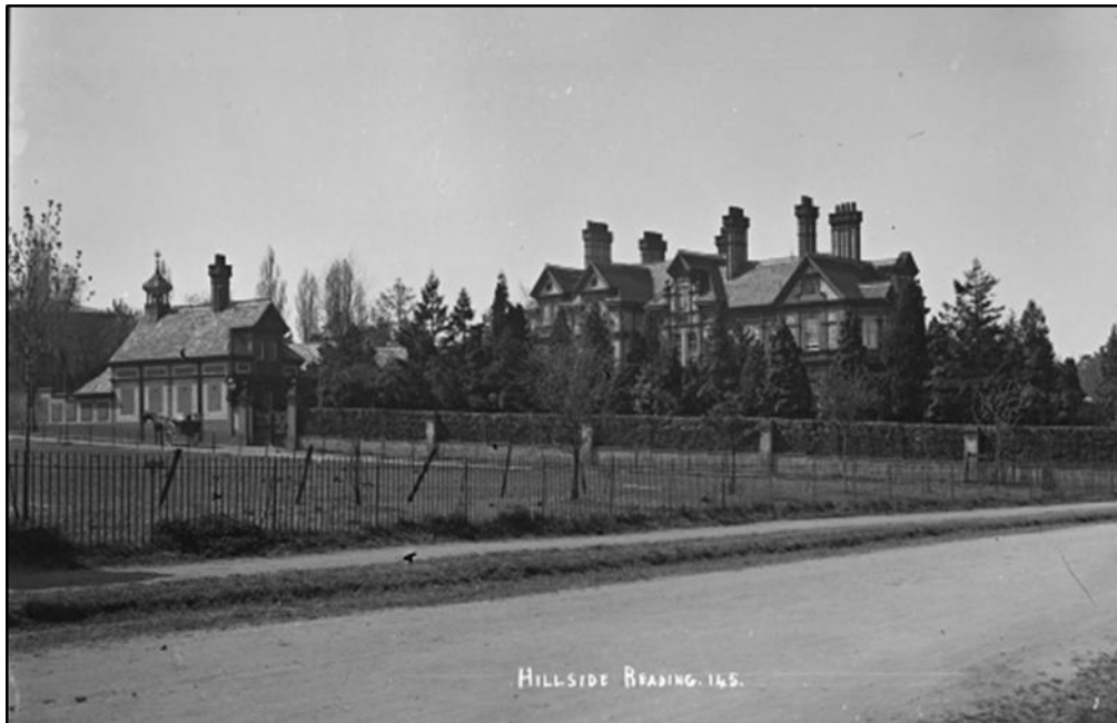
Figure 13 View of east elevation and Stable block. Courtesy of the Museum of English Rural Life
