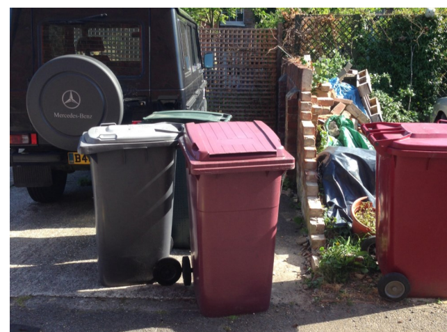
Boundary wall to rear of 142 and 140 Castle Hill
