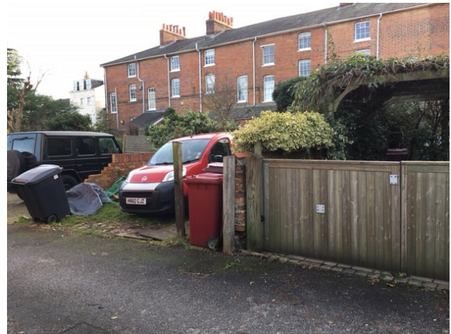
The rear of 142 Castle Hill, looking south east
