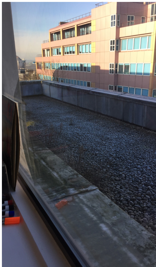
Existing 5th floor terrace overlooking Forbury Road
