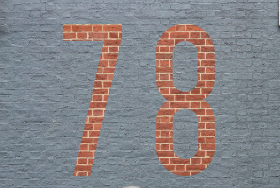
Building numbering in brick work
