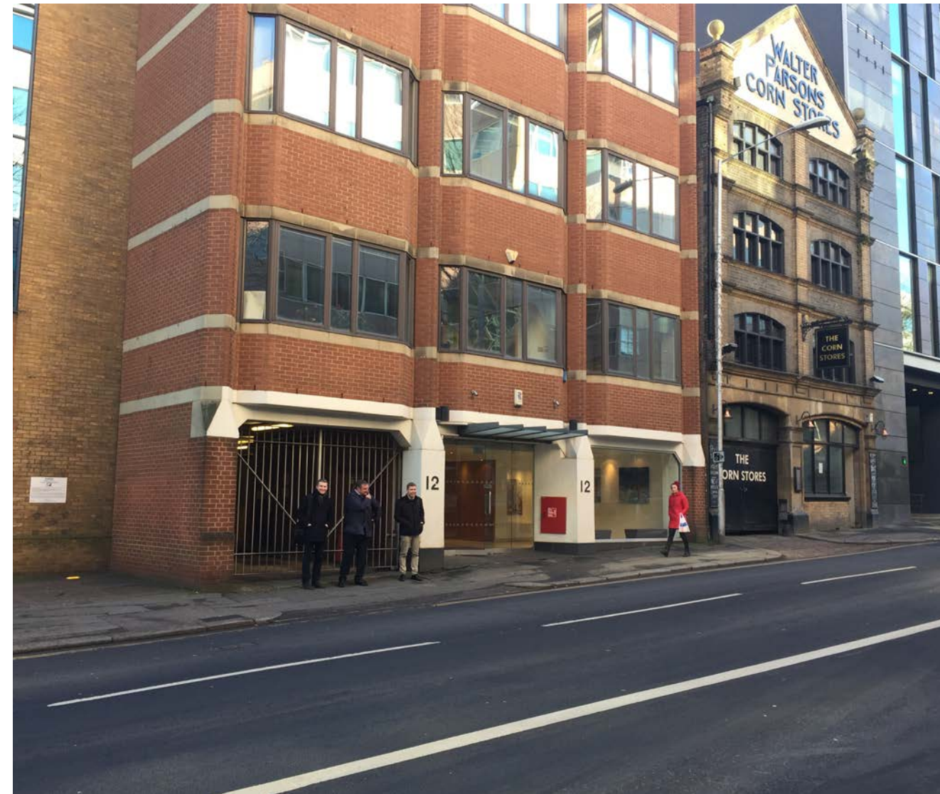
Forbury Court entrance on Forbury Road
