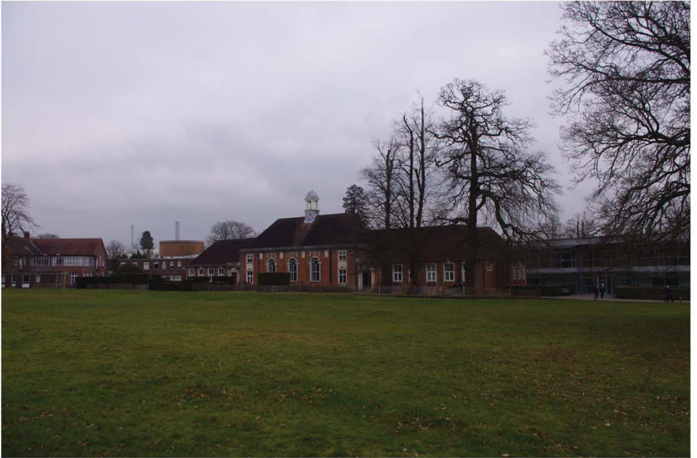
Plate 7 Peckover Hall, looking northeast
