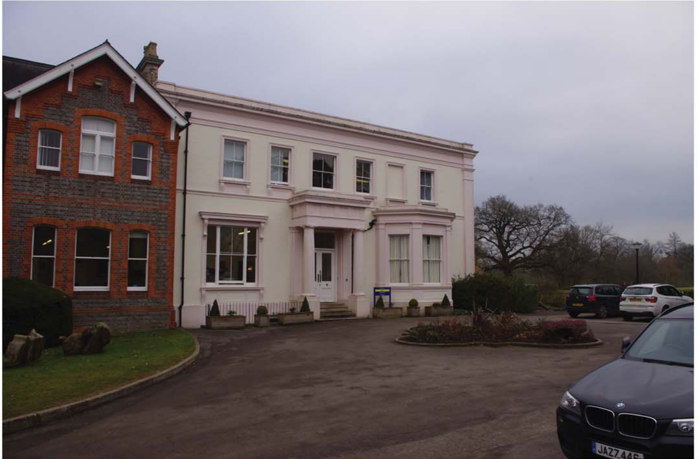
Plate 1 School House and attached Waterhouse laboratories, looking southeast
