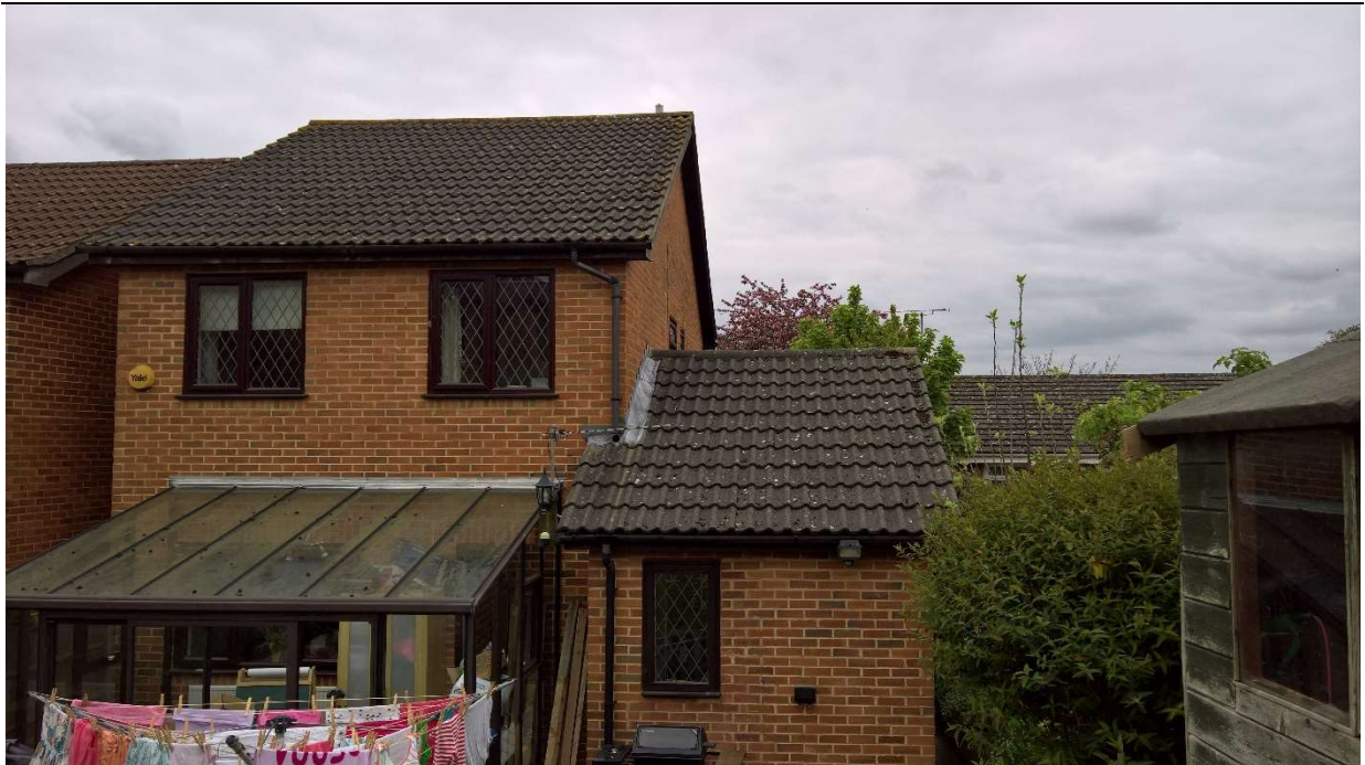
Rear Elevation (above) viewed from top of raised garden.
