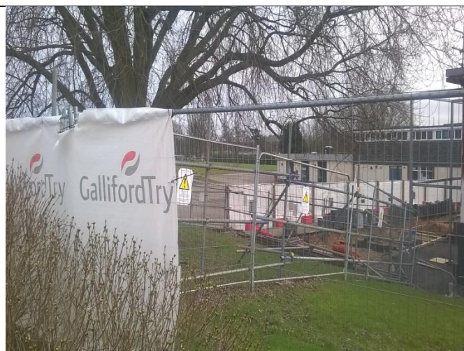
Herras fencing located around site, and in accordance with the approved method statement.
