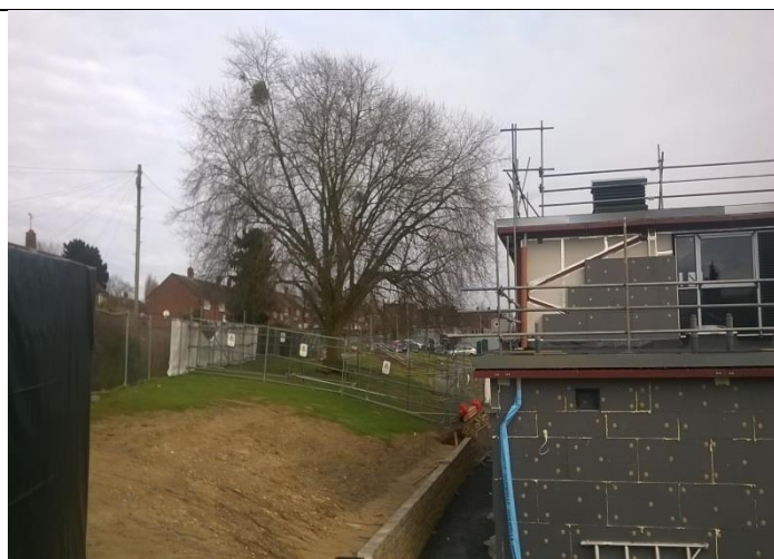
Herras fencing located around site, and in accordance with the approved method statement.
