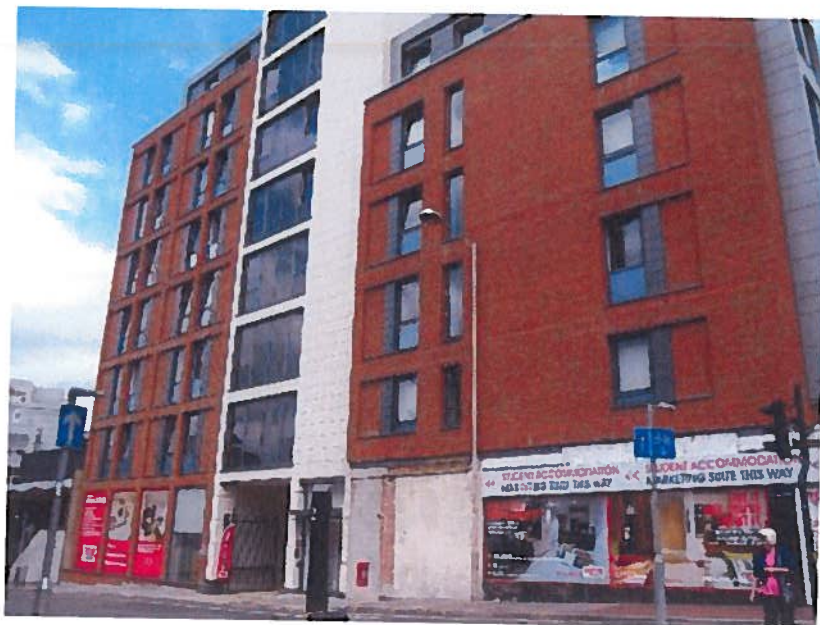
Photograph 2 – Front of adjacent building (Central Studios), showing gated entry to adjoining courtyard (view of west elevation, Greyfriars Road)
