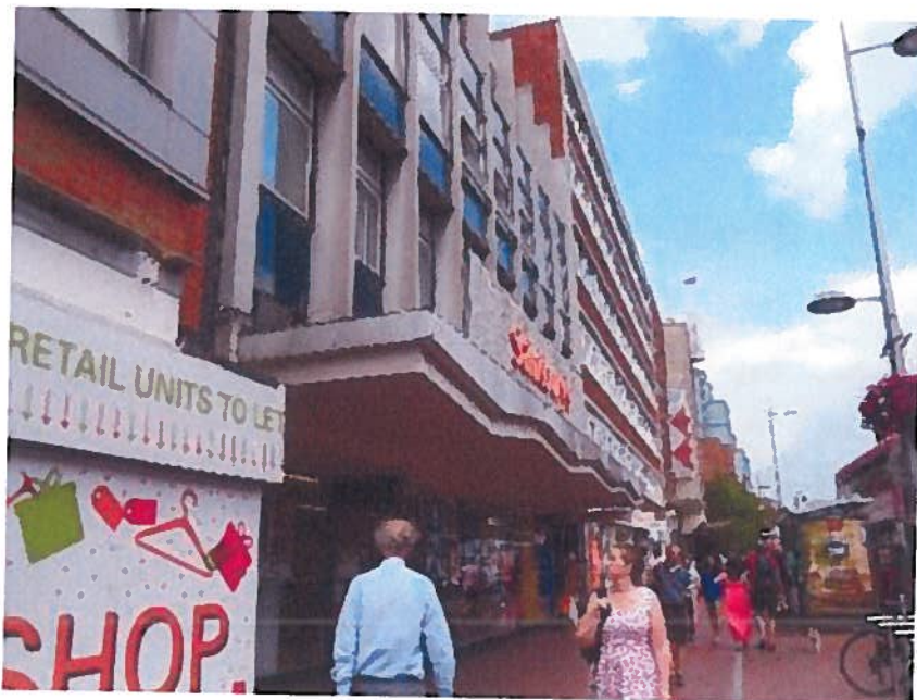
Photograph 1 - Front of building (south elevation, Friar Street)
