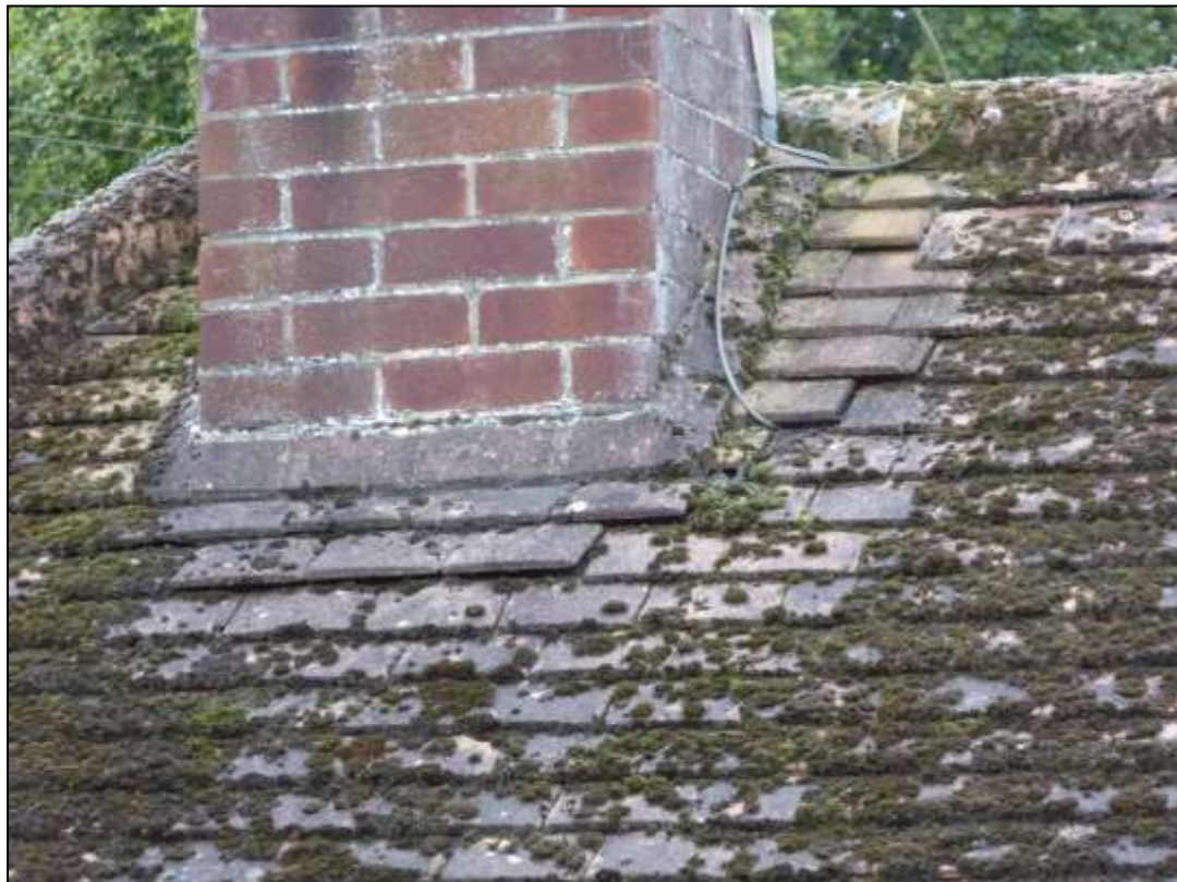
Figure 5. Gaps around chimney, 140 Kidmore End Road, Emmer Green. 06.10.16.
