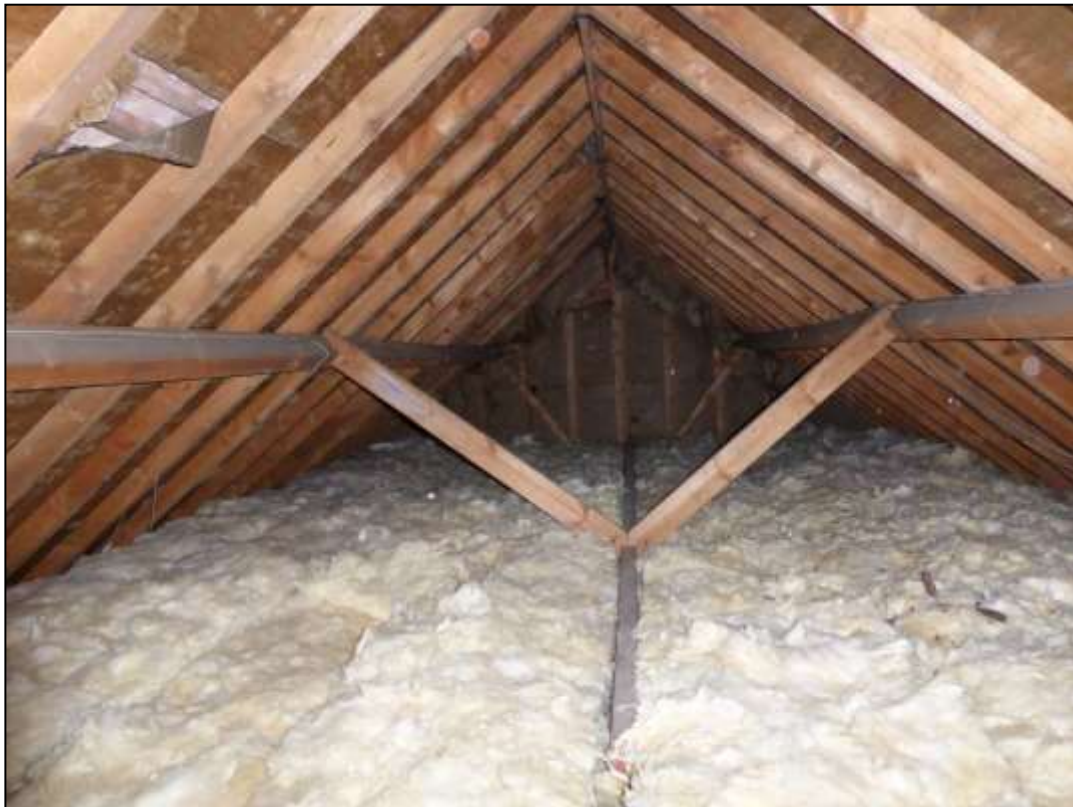
Figure 8. Example of loft space, 140 Kidmore End Road, Emmer Green. 06.10.16.
