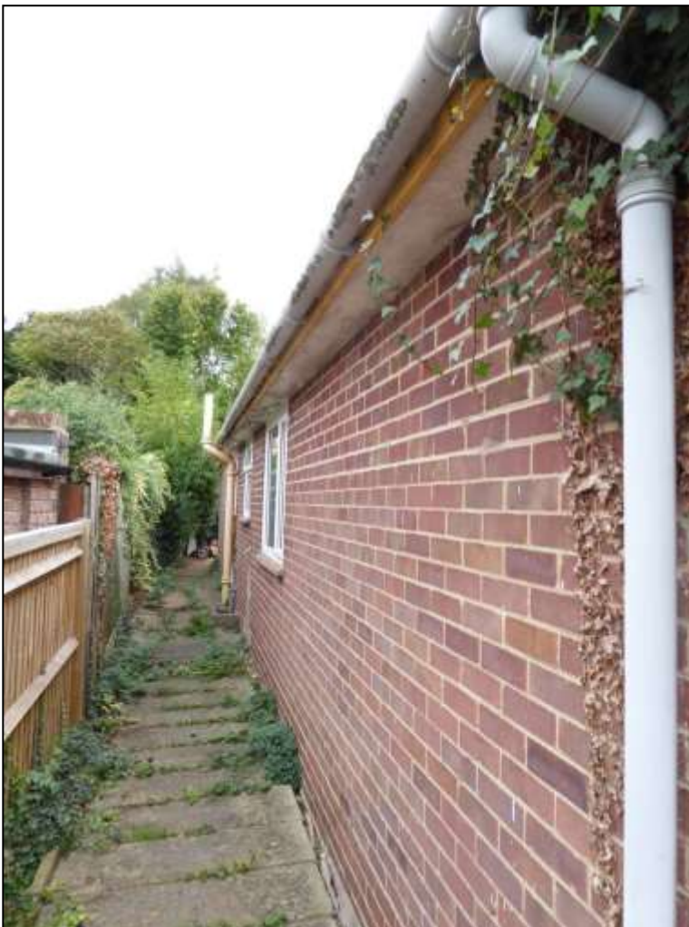
Figure 7. Example of soffits, 140 Kidmore End Road, Emmer Green. 06.10.16.
