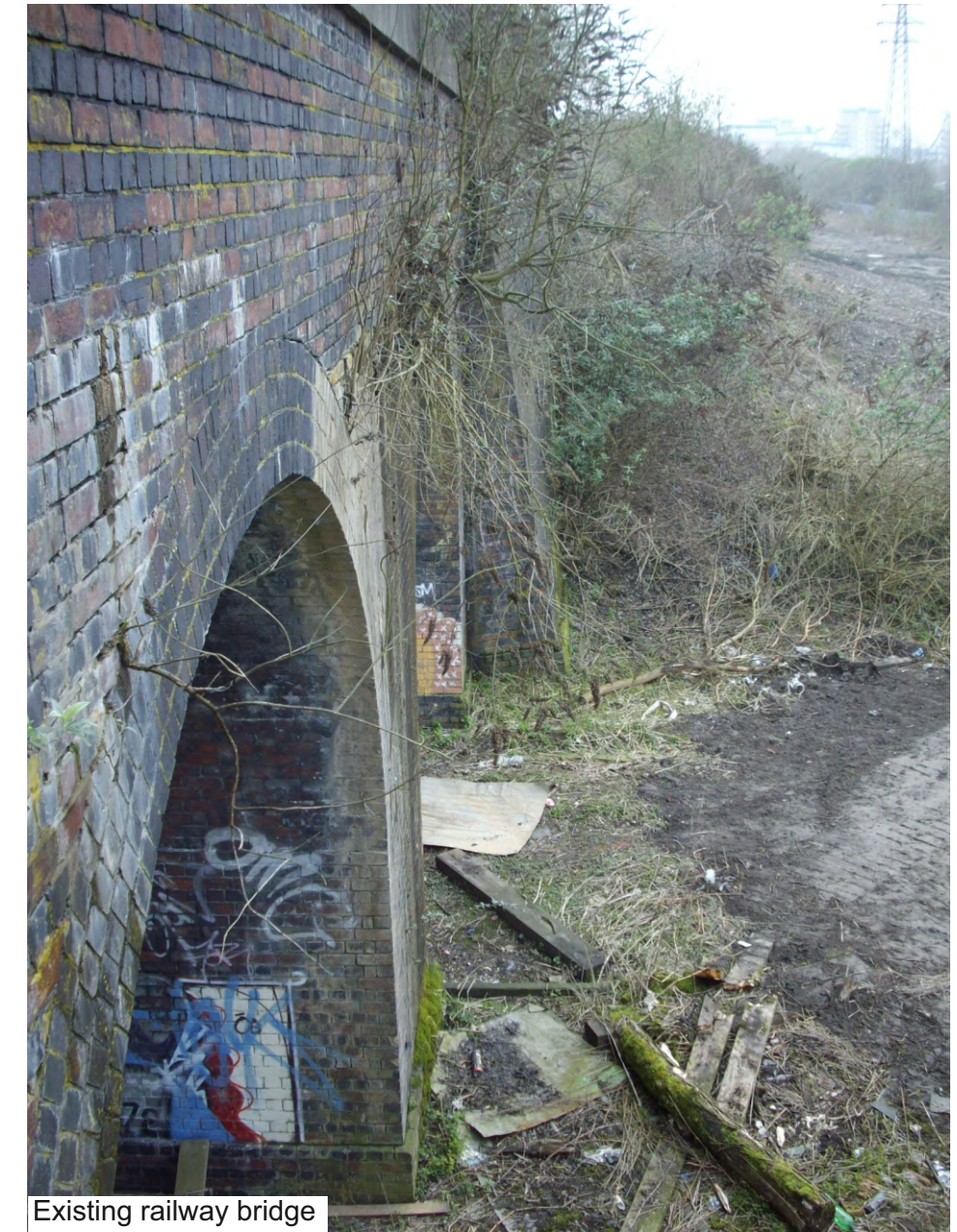
Existing railway bridge
