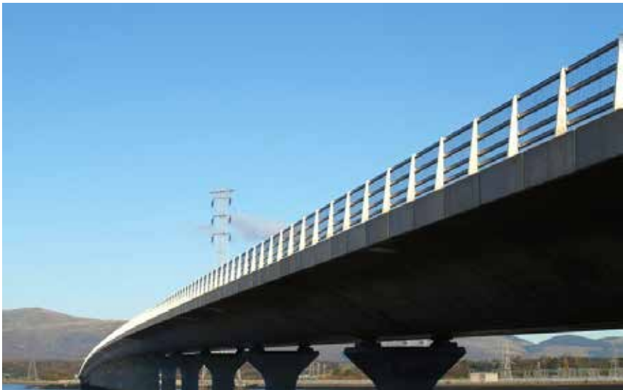
Figure 57. Example of railing with horizontal rails emphasizing curving form of viaduct
