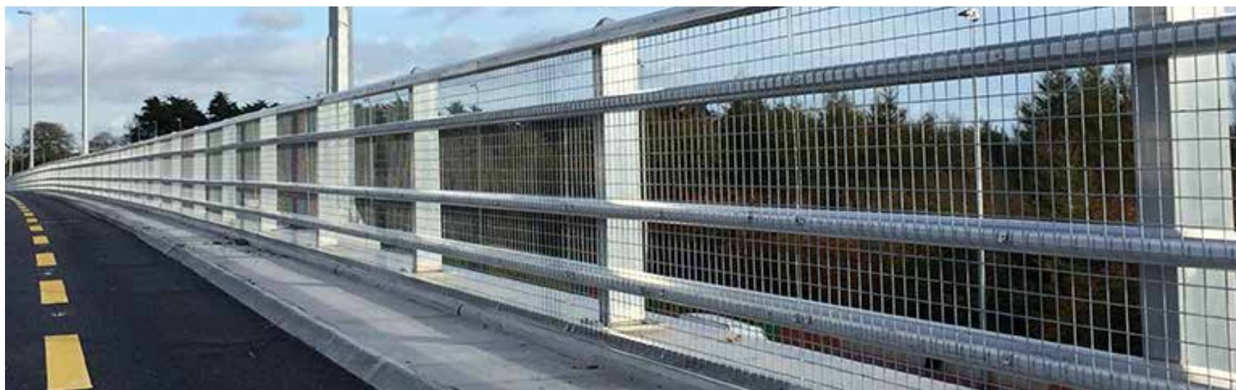
Figure 59. Balustrade rail with mesh infill
