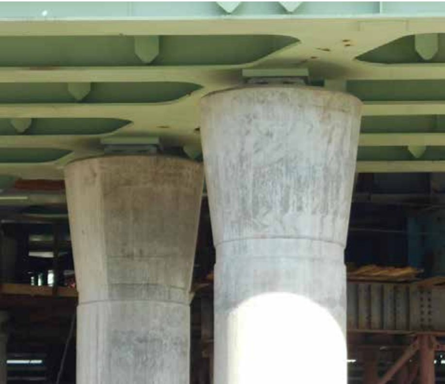
Figure 56. Example of tapered column head
