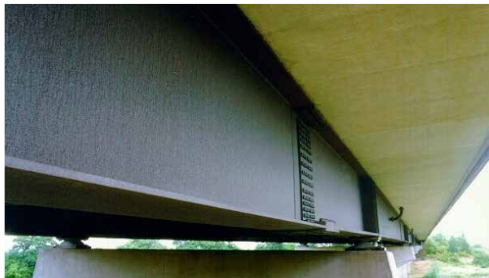
Figure 58. Example of weathering steel finish
