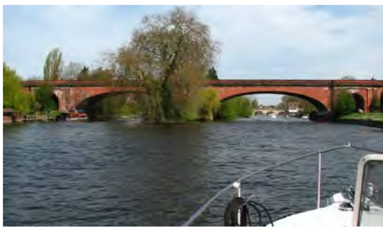
Figure 28. Maidenhead Railway Bridge
