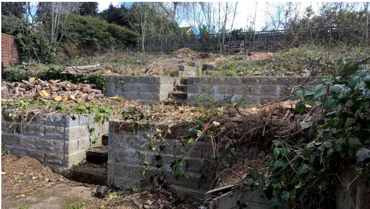
Garden tier retaining walls (Below).
