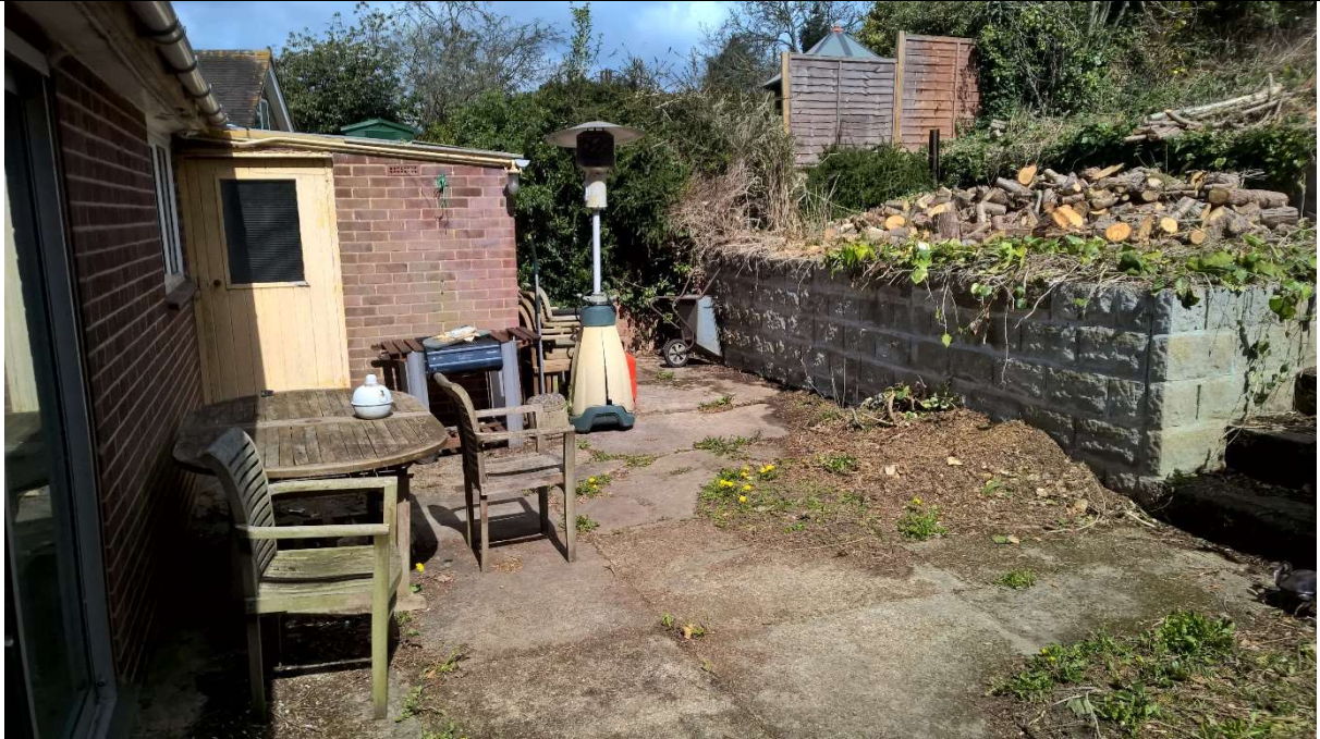
Existing lean-to extension (above).
