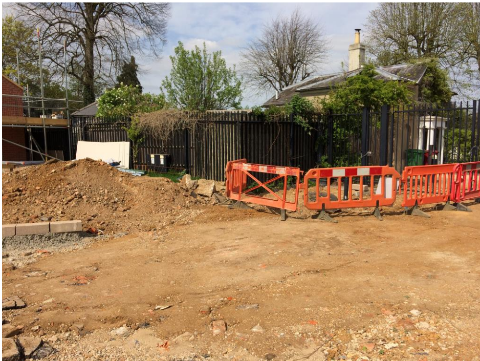
Plate 7: View of West Lodge as seen from the current construction area to the south east.
