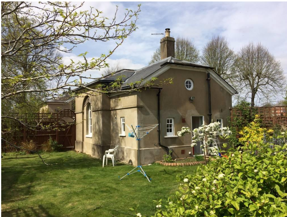
Plate 2: South and east elevations of East Lodge as seen within the garden areas to the southeast.
