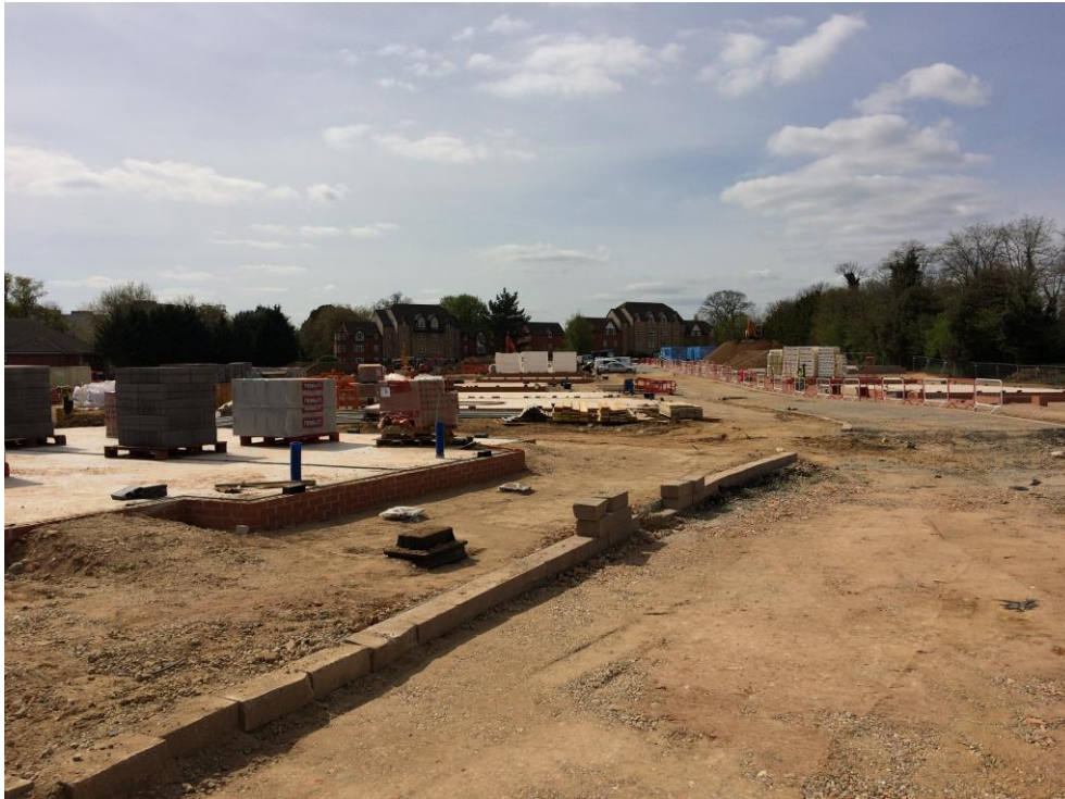
Plate 8: View west across the current construction works to the west of the Lodges.
