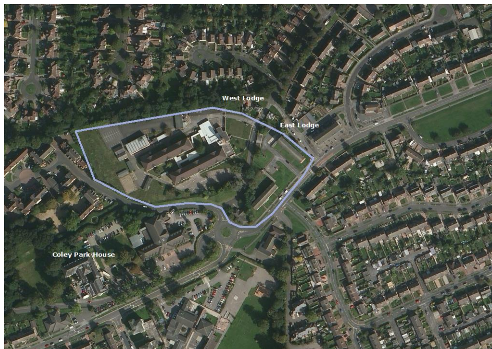
Plate 5: Aerial photograph of East Lodge and its surrounds. Note that the area in purple is currently being redeveloped.
