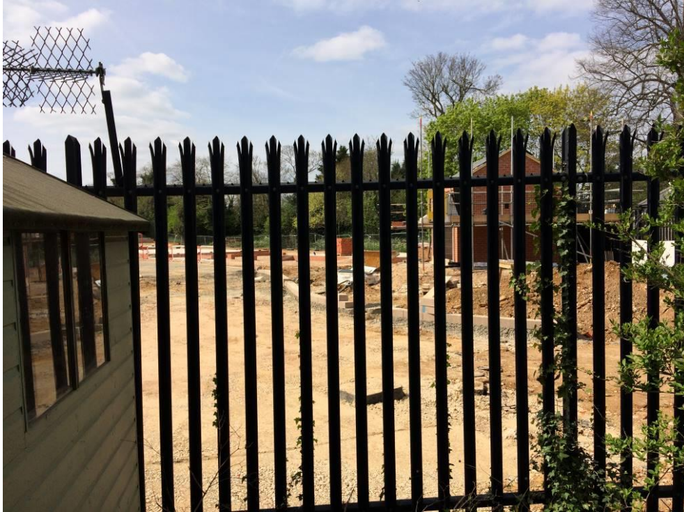
Plate 6: View northeast from the area of the proposed outbuildings towards current construction area.
