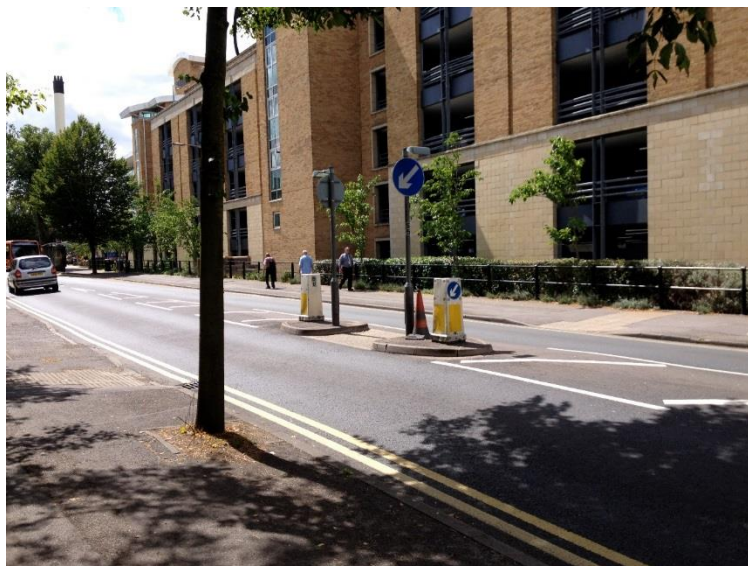
Photograph 4: Pedestrian Refuge Island on Craven Road
