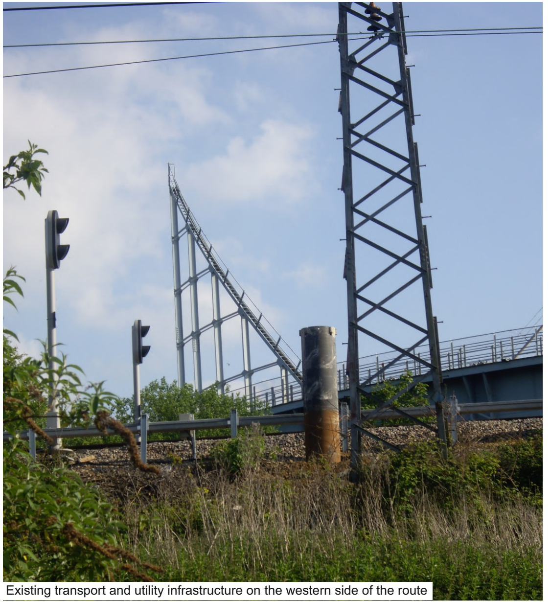
Existing transport and utility infrastructure on the western side of the route
