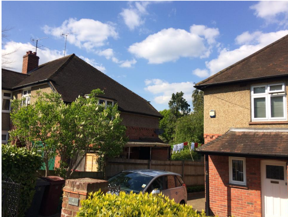
Side facing window and lean-to car port of no.6
