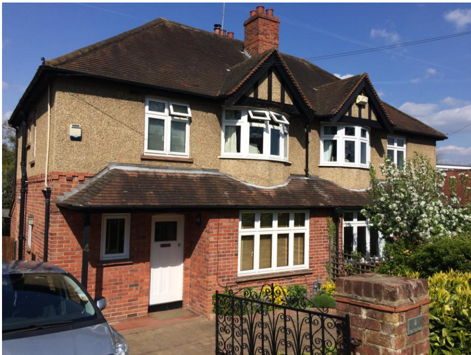
Existing front elevation of property
