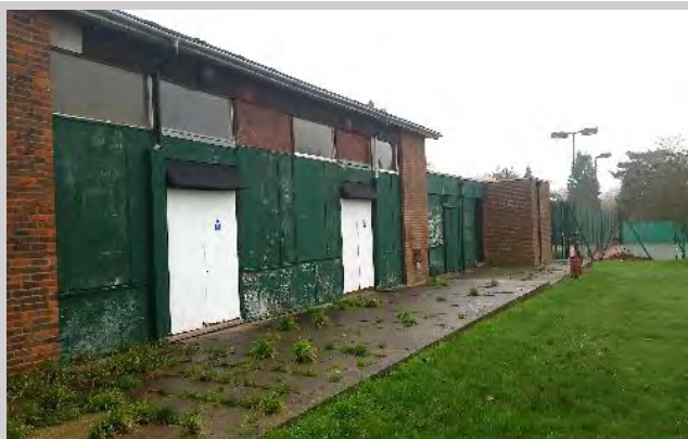
Photo 1. Building 1, south face looking north-east.
