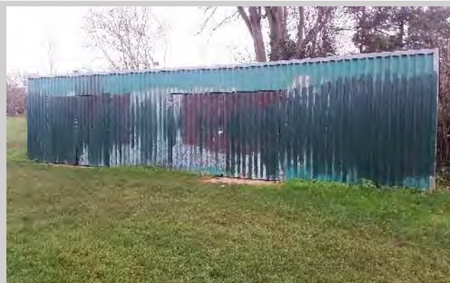
Photo 2: Building 2, south face looking north.
