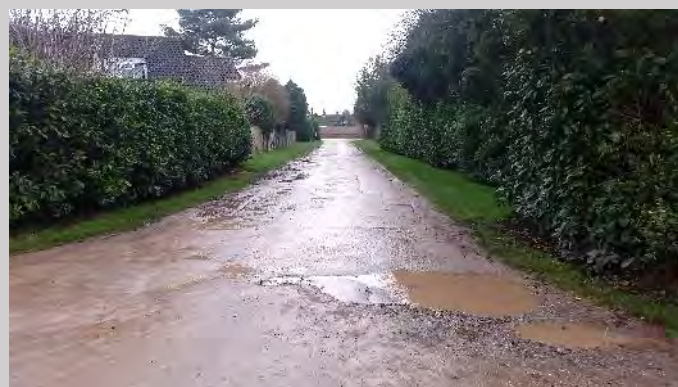
Photo 7: Northern site entrance.
