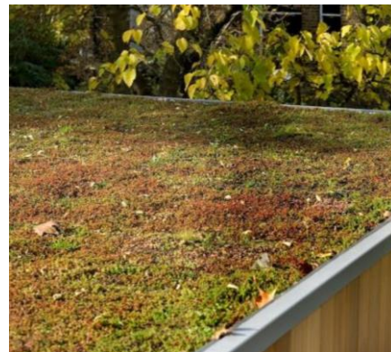
Clear treated hardwood fascia with aluminium capping - sedum planted roof finish
