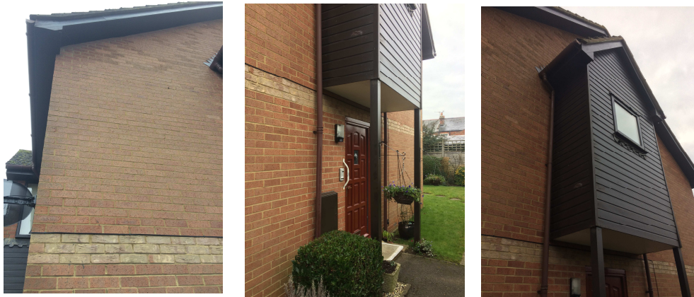
Photo 4: External West Facing Elevation (Rear of the Main block with 16 dwellings)
