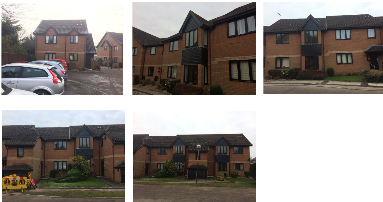
Photos 2: East Facing External Elevations (Main block with 16 dwellings)
