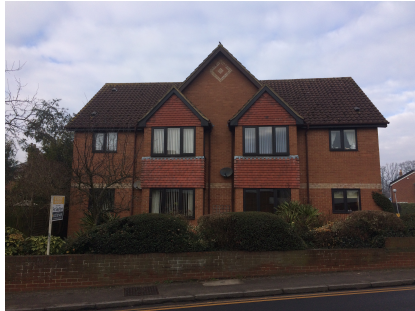
Photo 6: External North Facing Elevation (Rear of the Main block with 16 dwellings)
