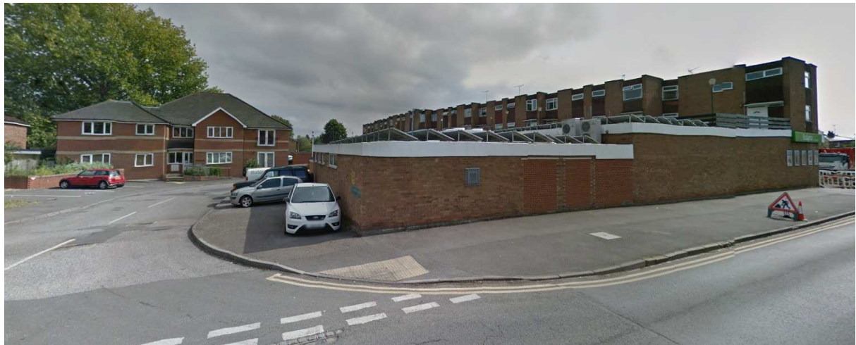
Photo 7: Existing properties adjacent to site with PVC-u windows.
