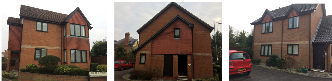
Photos 1: Existing External Elevations – Two Semi-Detached Dwellings
