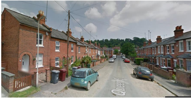
View down Queen Street showing two bedroom terraced houses
