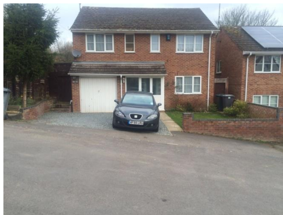
The existing house
