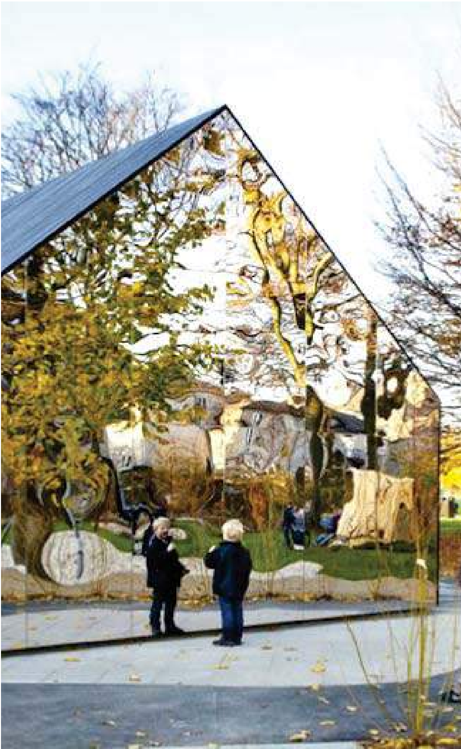
Substation / Bin&Bike store (facing LEAP) polished stainless steel precedent
