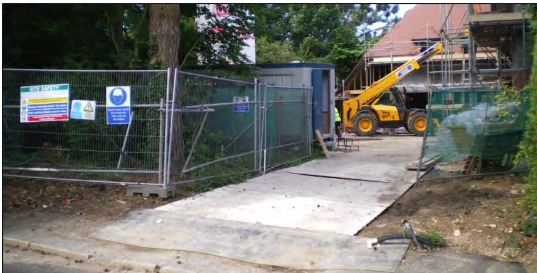
Vehicular ground protection trackway
