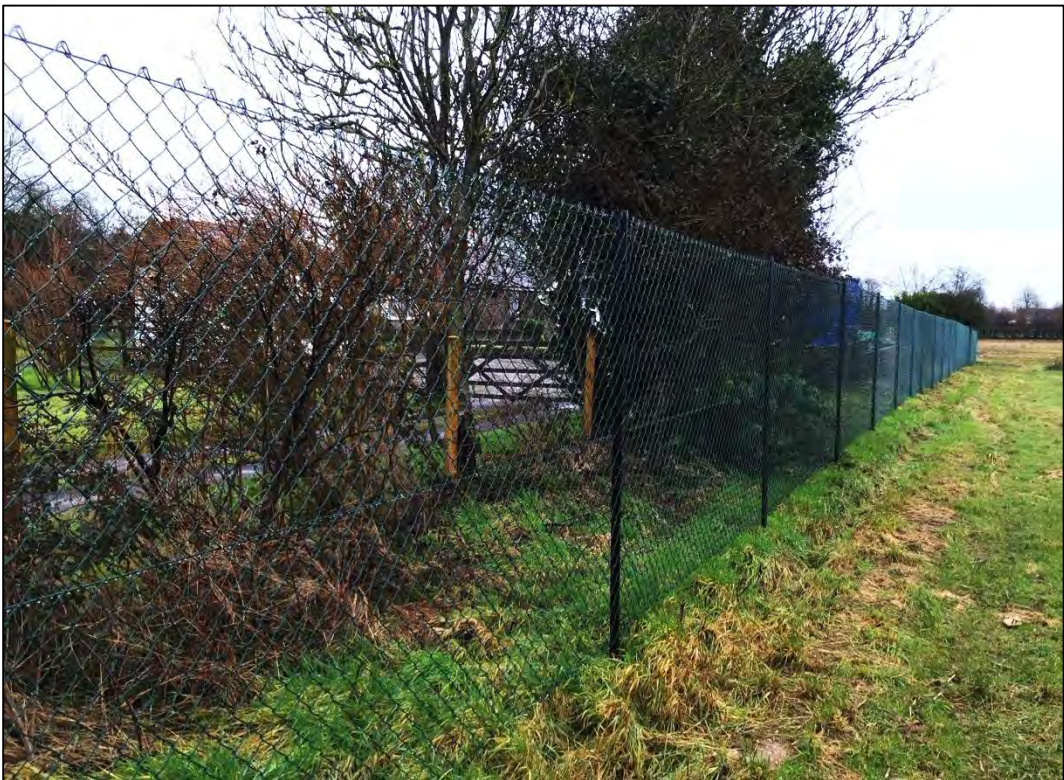
Chain-link on angle-iron uprights
