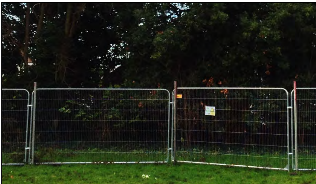
Weld-mesh panels on scaffold uprights
