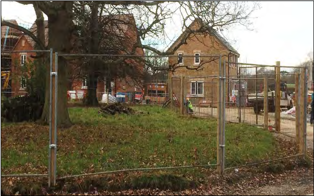
Weld-mesh panels on wooden posts
