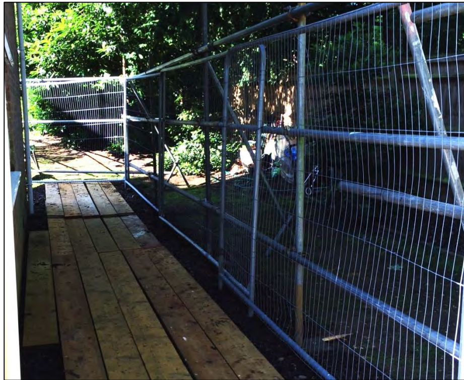
Scaffold board pedestrian ground protection
