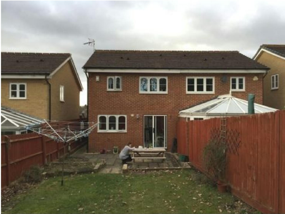
Photo02: Rear Elevation. To be extended
