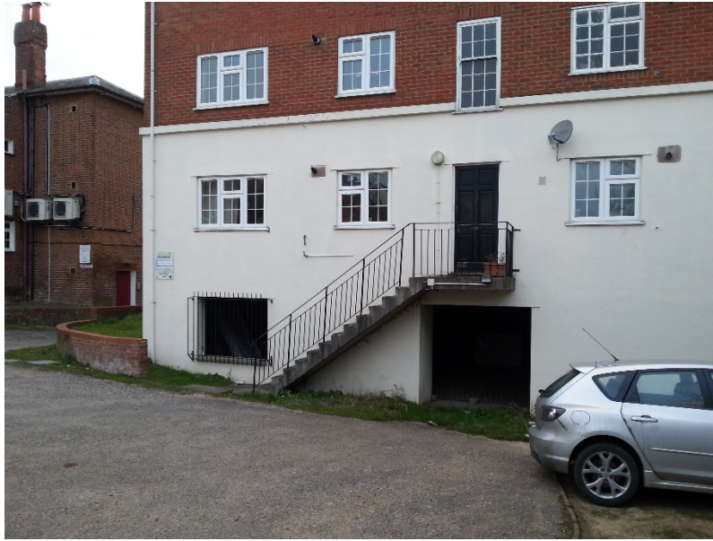
Fig. 4 – Photo from rear of property
