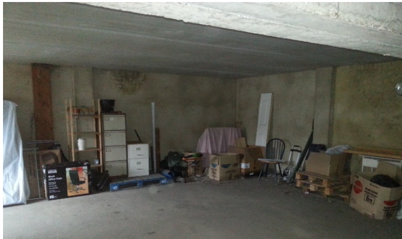
Fig. 5 – Photo inside basement
