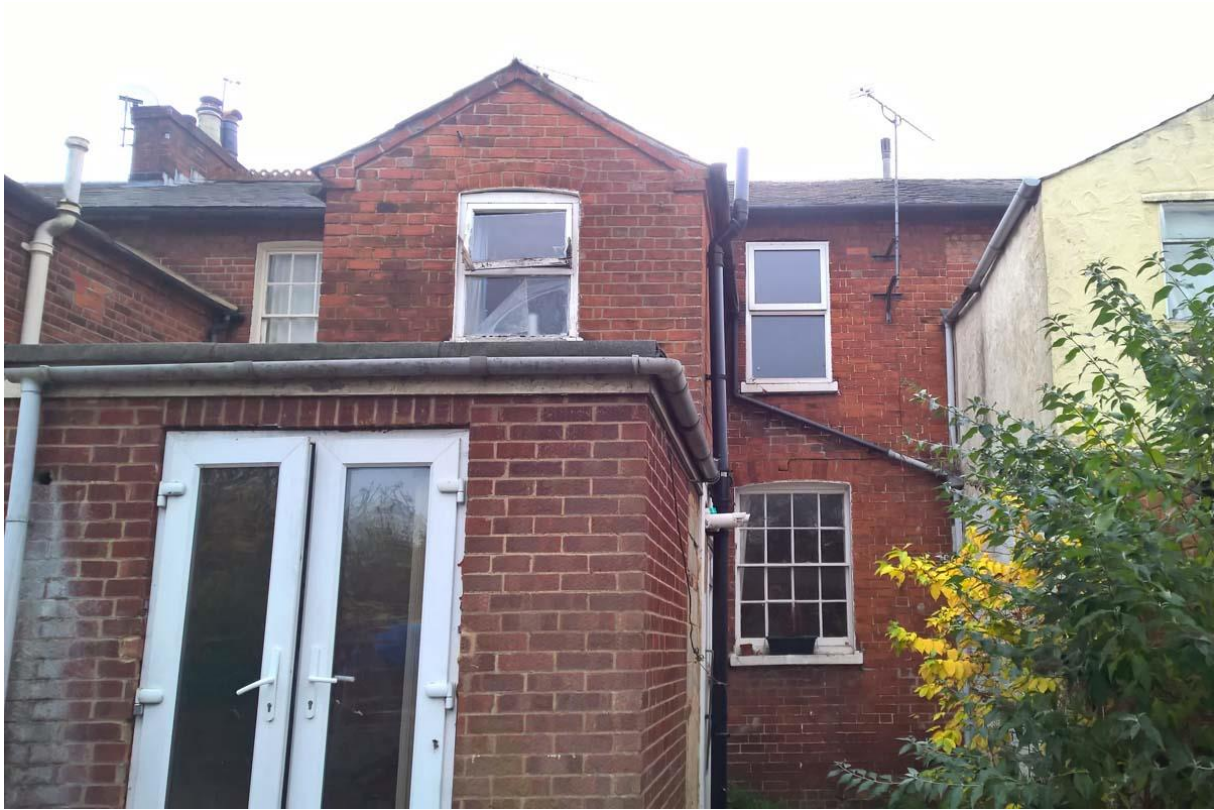
Modern rainwater goods to the North and West elevations
