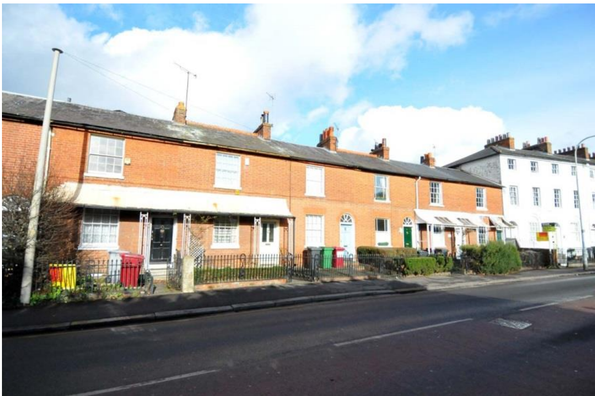
15 Christchurch Road, South elevation
