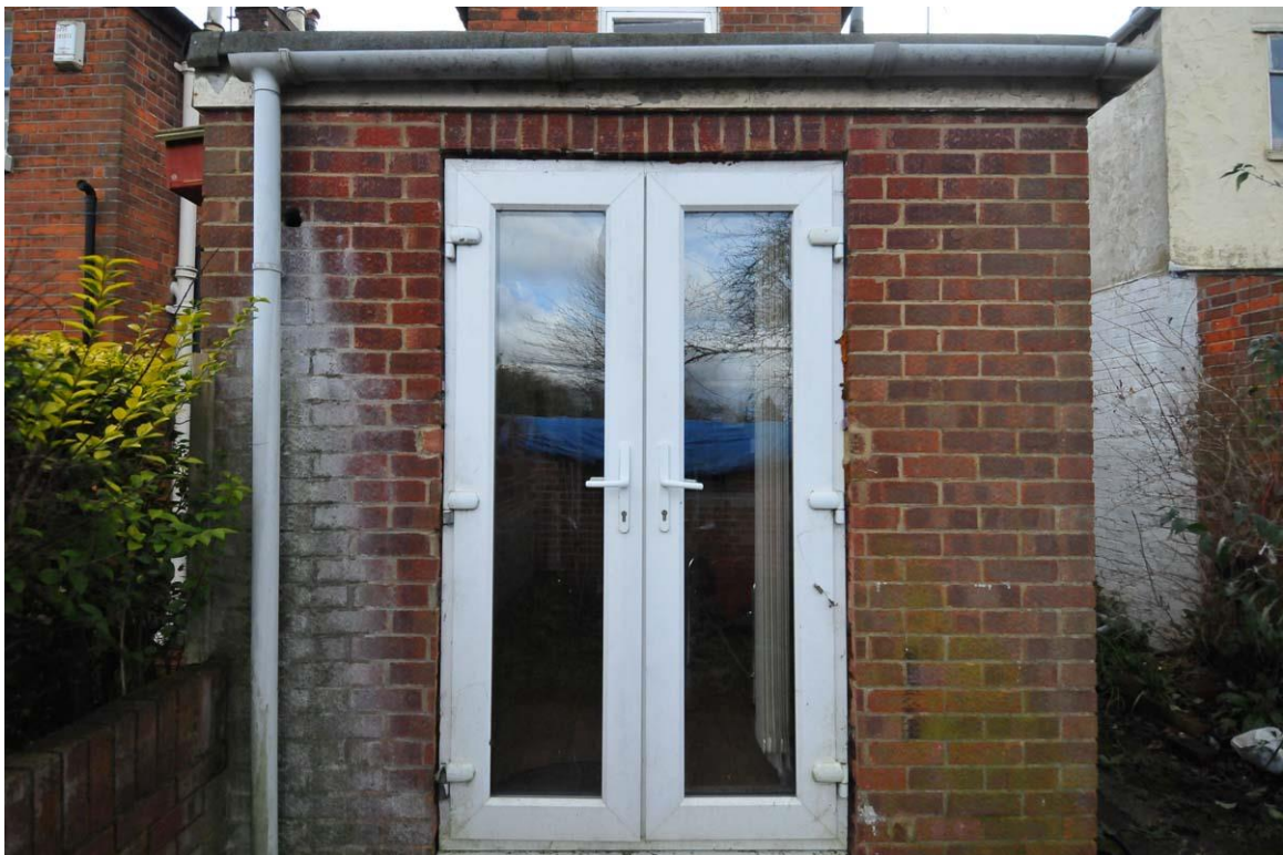
Existing doors, North elevation
