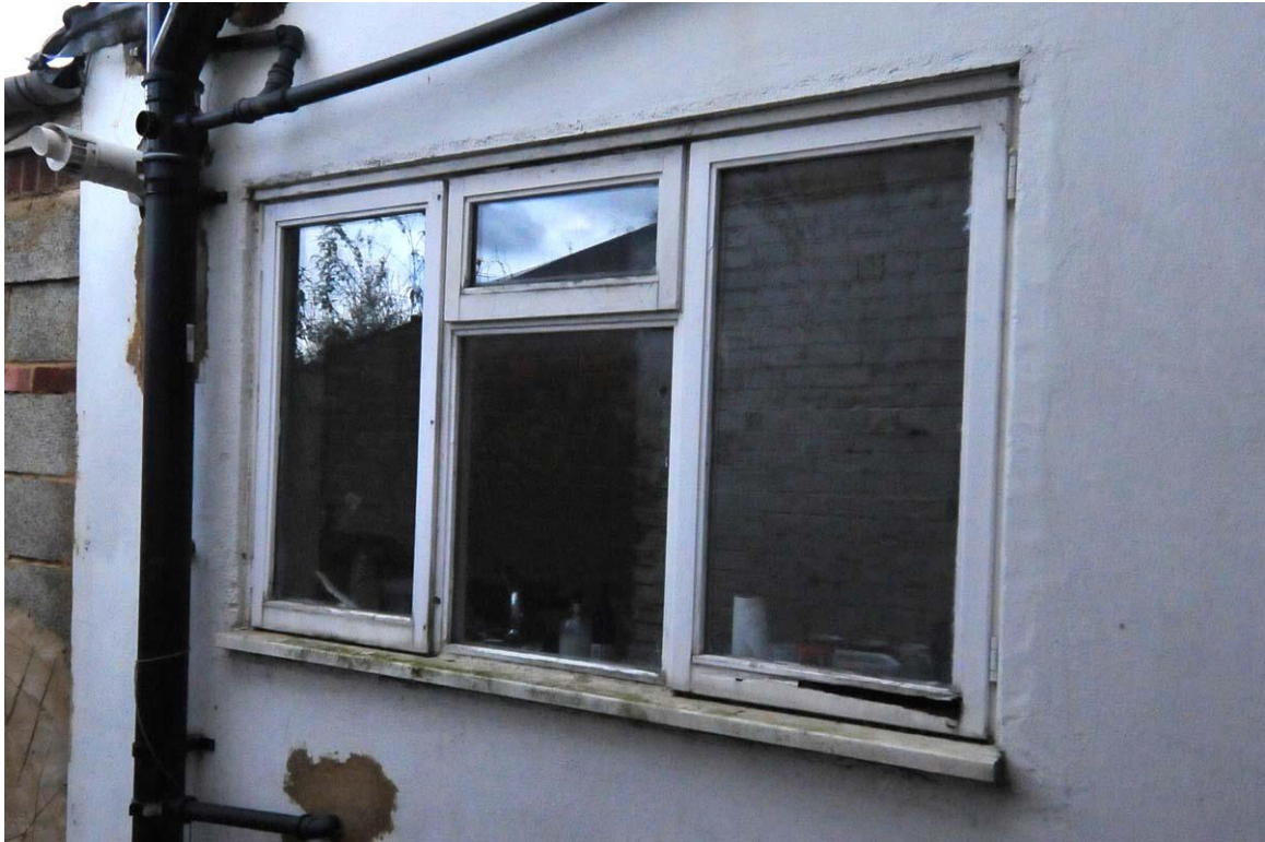
Existing window, West elevation
