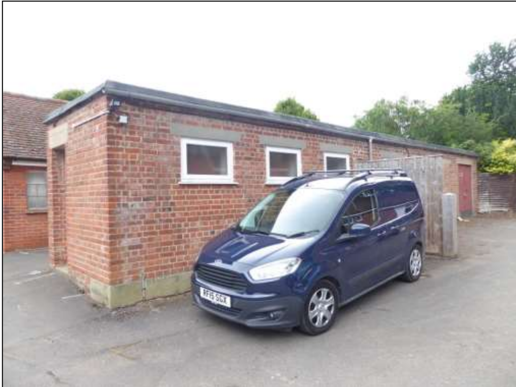
Figure 9. Example of store room construction, Henley Road Cemetery, Caversham. 03.07.17
