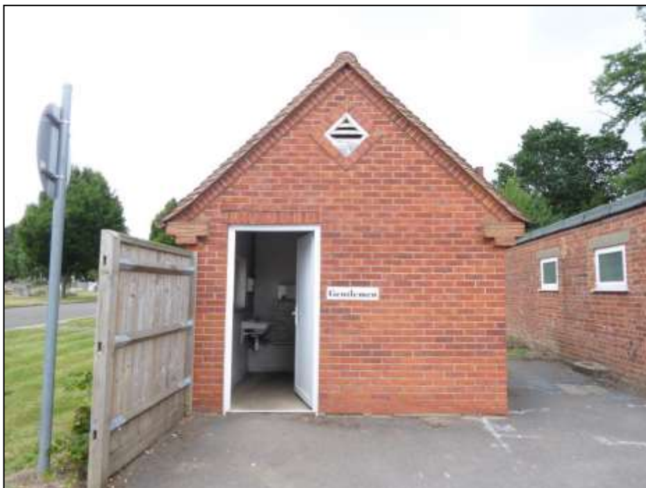
Figure 3. Front view of the toilet block, Henley Road Cemetery, Caversham. 03.07.17
