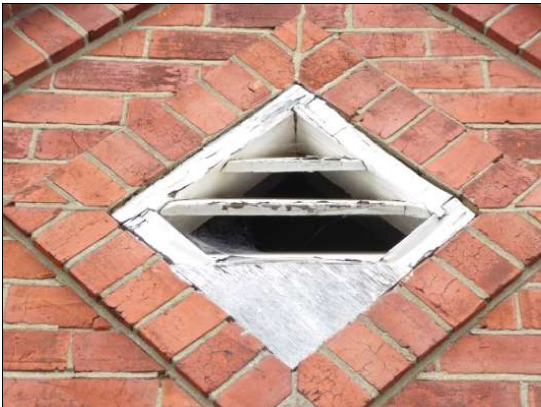
Figure 8. Example of louvered panels. Henley Road Cemetery, Caversham. 03.07.17
