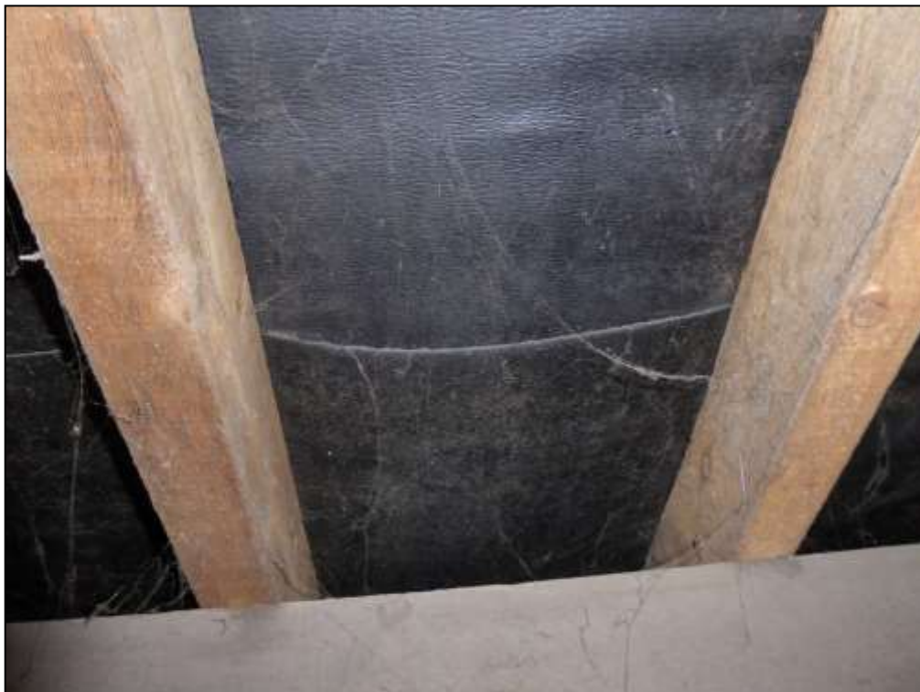
Figure 11. Example of bitumen lining, Henley Road Cemetery, Caversham, 03.07.17
