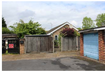
Adjacent Bungalow and Access
