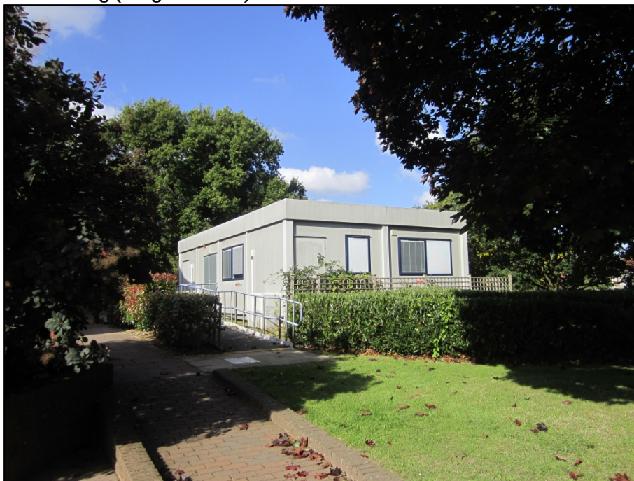
Plate 6. Demountable building (Target Note 2)
