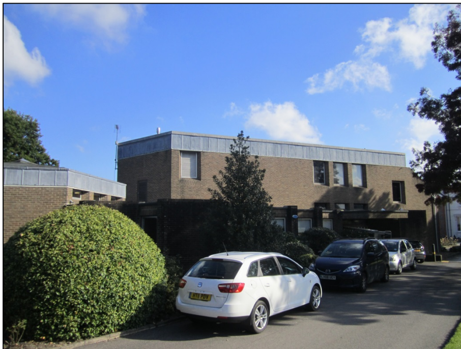
Plate 4. Two storey brick building (Target Note 1, viewed towards southern elevation)
