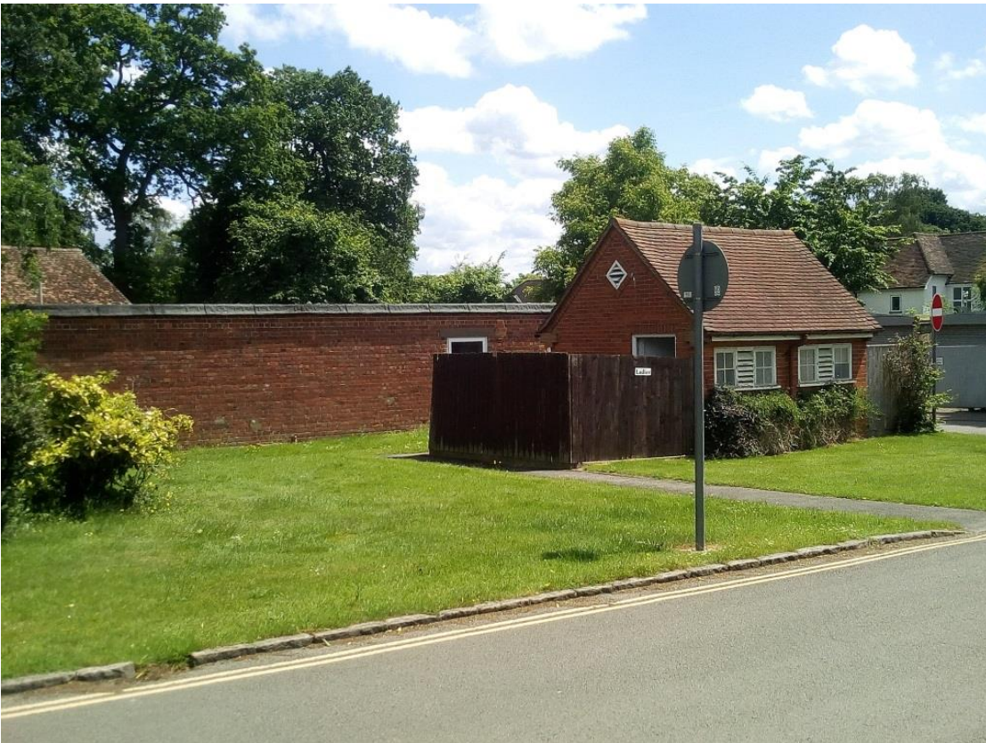
View of development site from the North West
