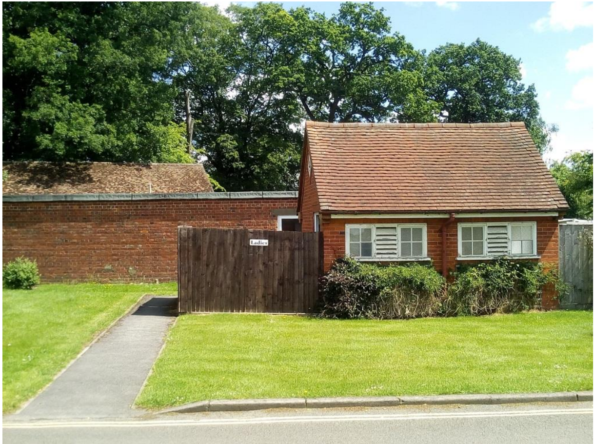
Toilet Block with Grounds Maintenance Store behind (to be demolished)
