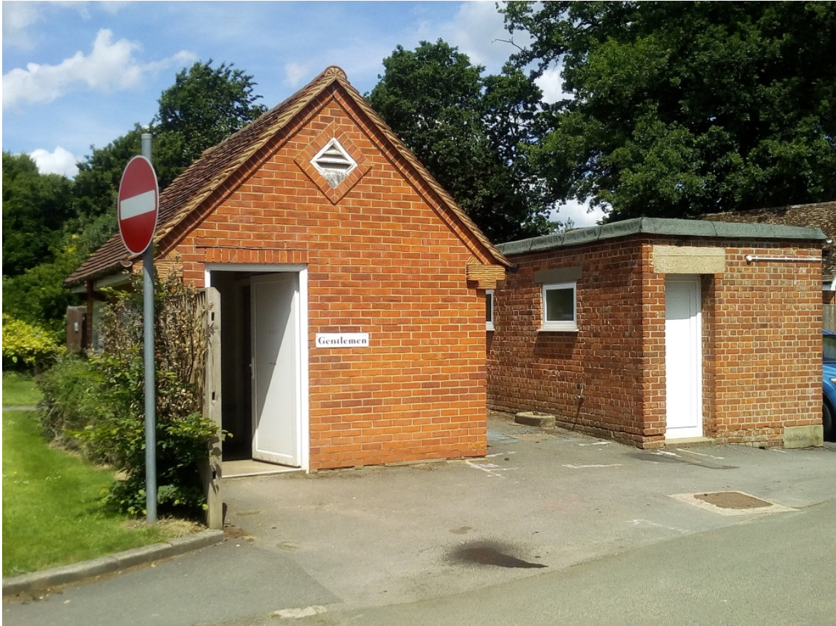
Toilet Block and Grounds Maintenance Store (to be demolished)
