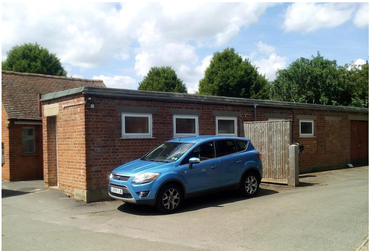
Grounds Maintenance Store (to be demolished)
