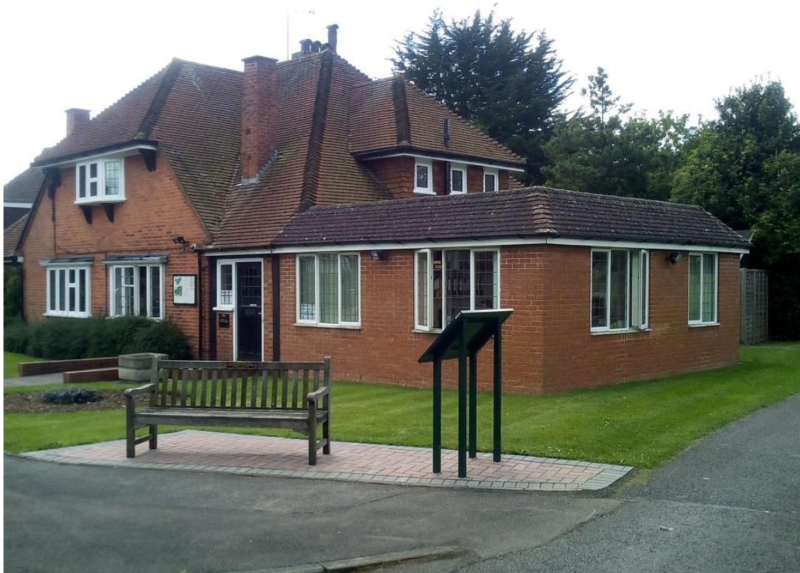
Existing Office & Lodge (to be retained)
