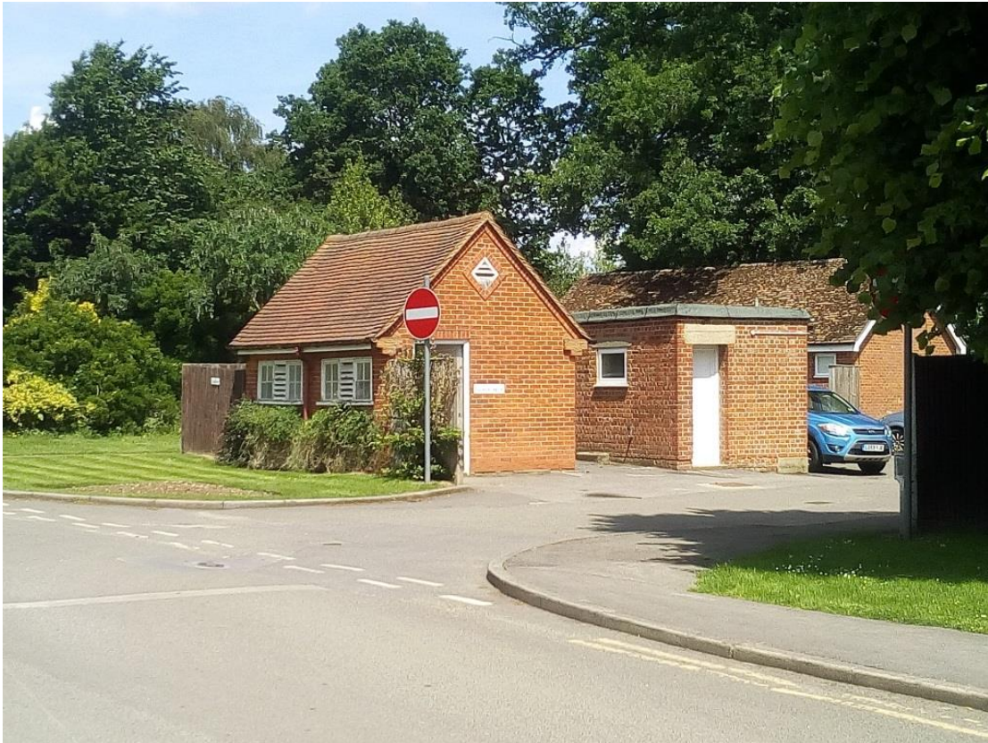
View of development site from the South
