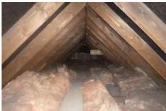
7. Roof space showing fibreglass floor insulation and newly fitted felt.
