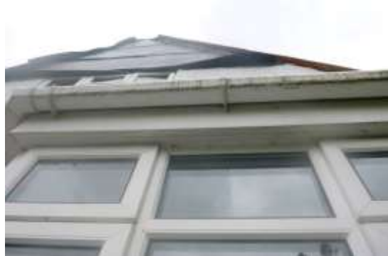
6. Tightly fitted soffits around the ground floor dormer window to the front of the house.
