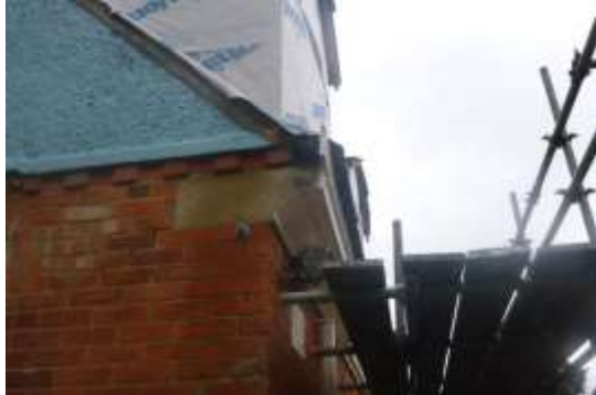
5. Tightly fitted soffits below the new dormers.
