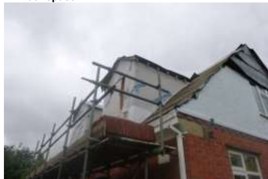
4. Newly constructed dormers to the side of the property and the removed roof tiles.
