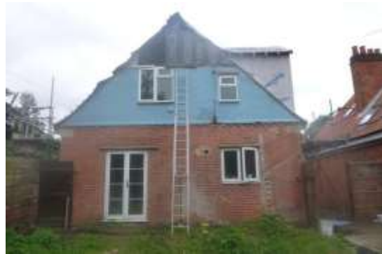
2. Rear views of the house showing the newly constructed dormers and access point to the roof space.
