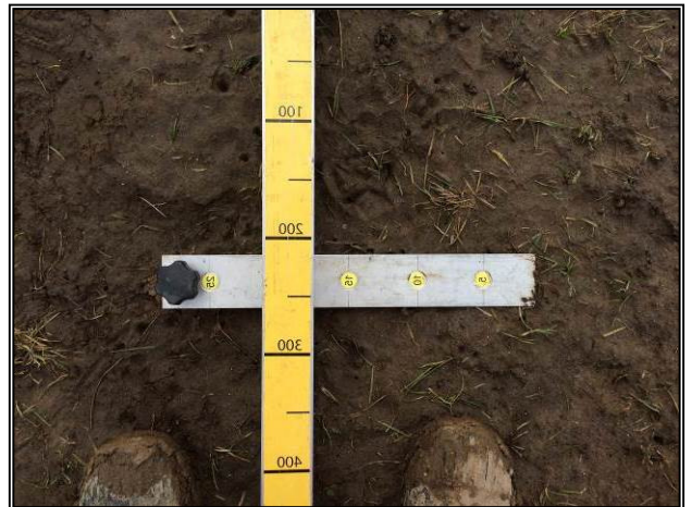
Plate 20: Significant undulation – 21mm measured using wedge under 3 metre straight edge
