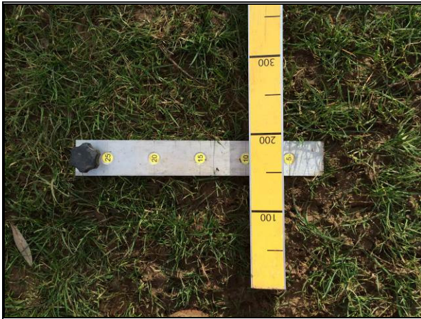
Plate 19: Minor undulation – 7mm measured using wedge under 3 metre straight edge
