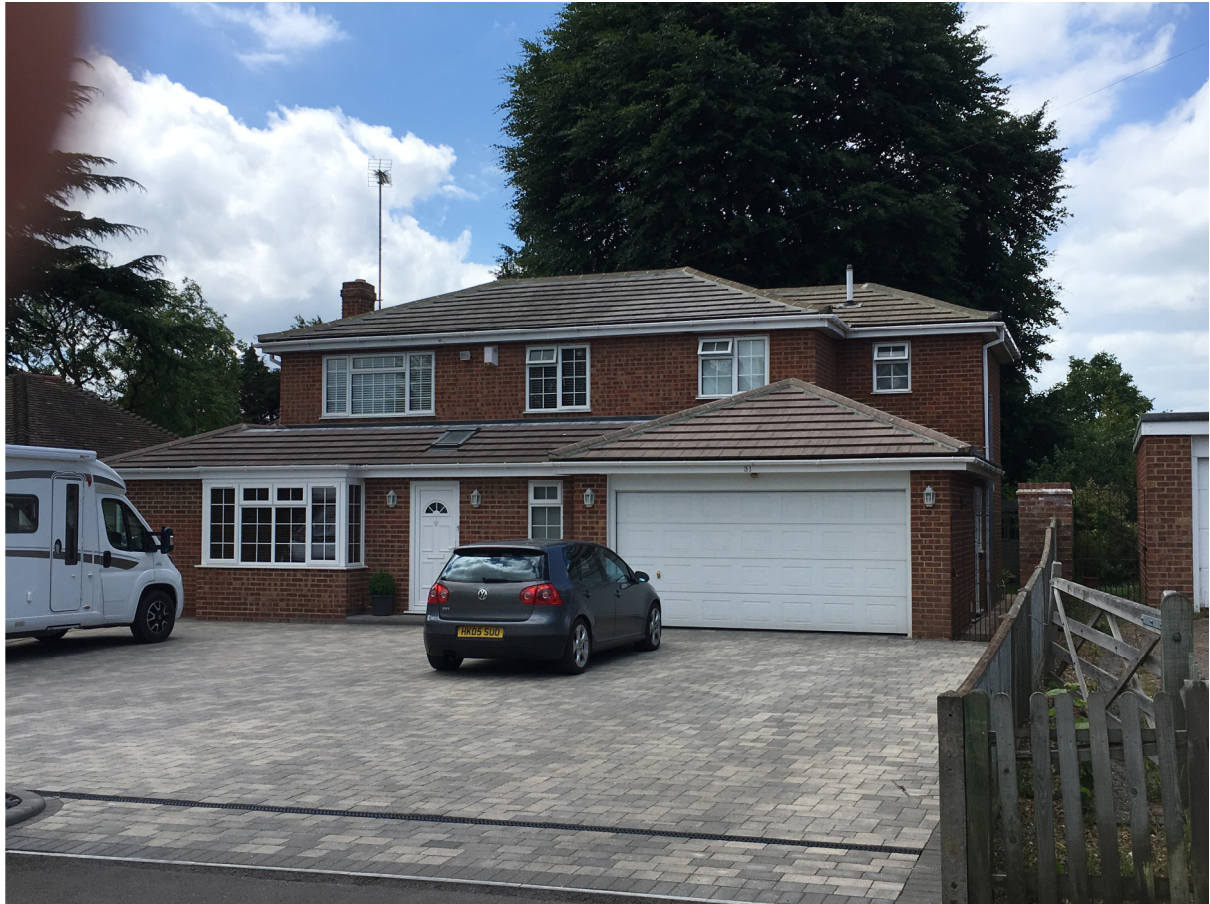
Photograph of a similar completed extension at the neighbouring no. 31, Conisboro Avenue Similar construction to our proposal at No 31 Conisboro Avenue
