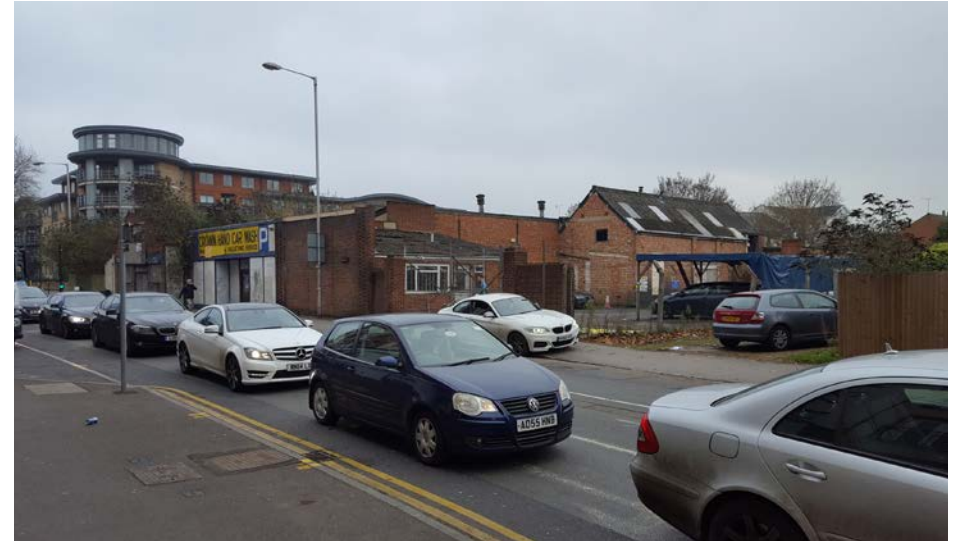
Photo: Existing brickwork buildings on Site looking from opposite side of Crown St
