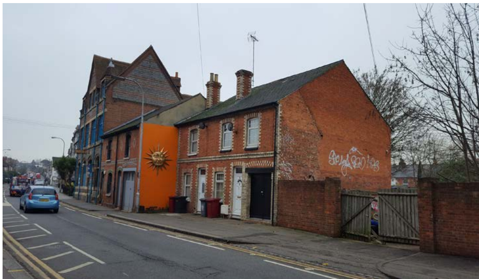
Photo: View of existing Silver St site access, on right, with gable of 22 Silver St and former Rising Sun Temperance Tavern beyond
