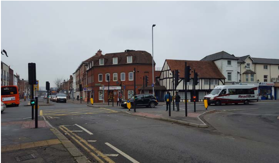
Photo: View of 3-5 London Road (timber-framed) with 7-11 London Road to their right
