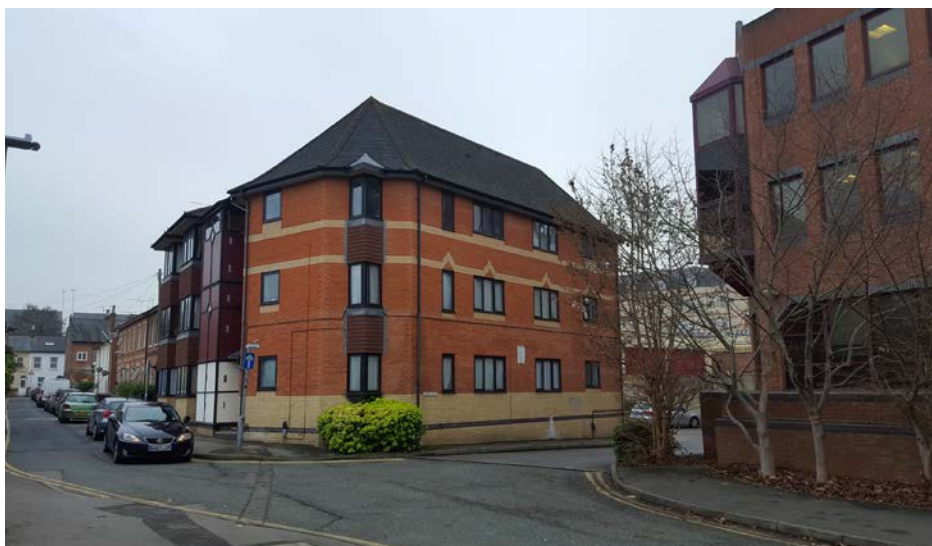
Photo: View of 1-14 Priors Court from north
