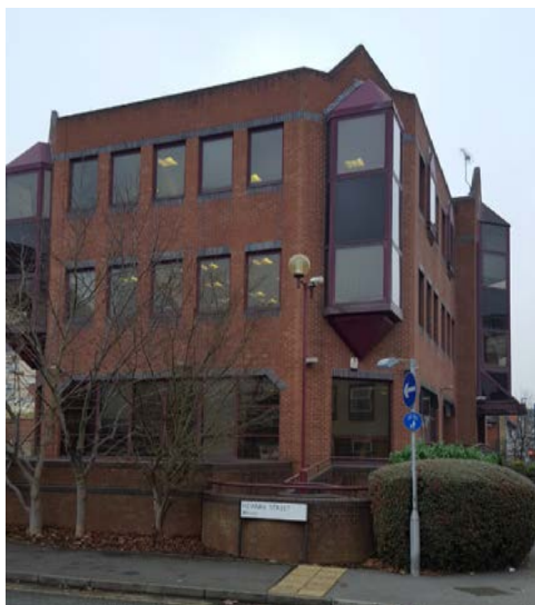
Photo: View of Regents Gate from east
