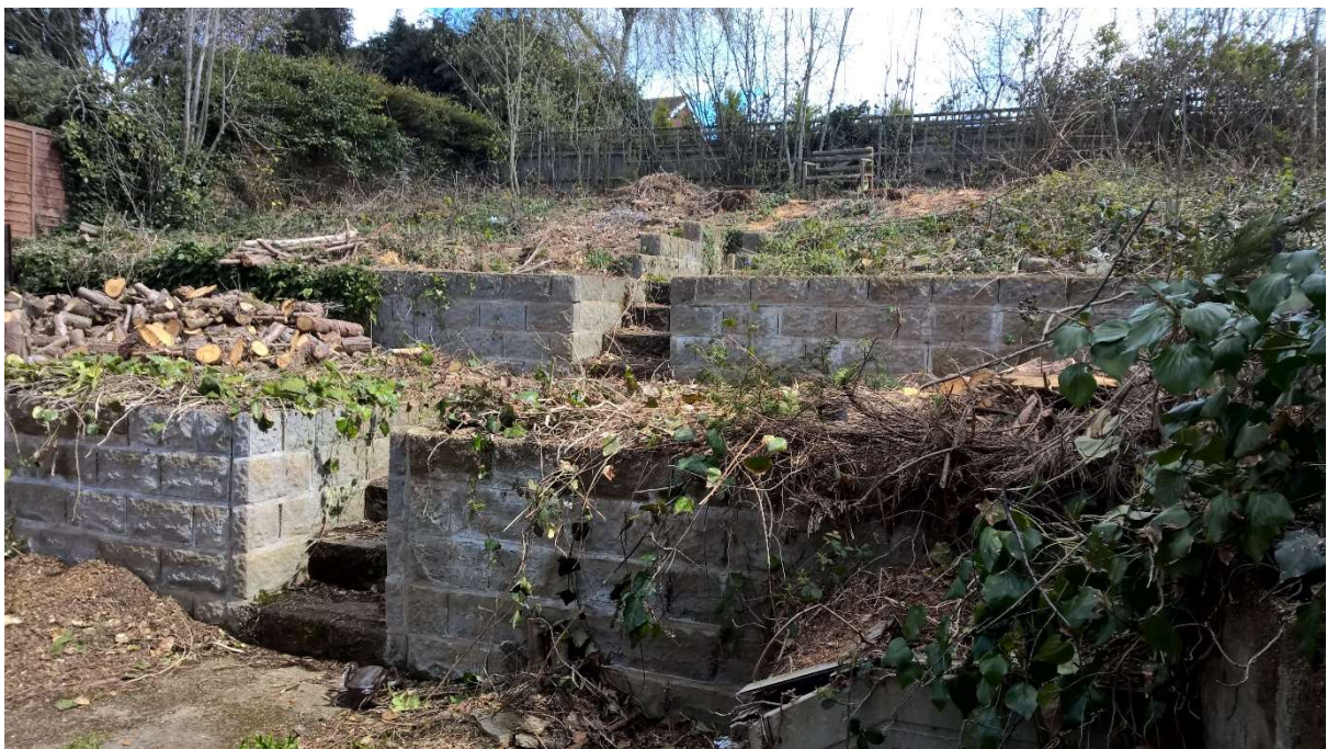
Garden tier retaining walls (Below).
