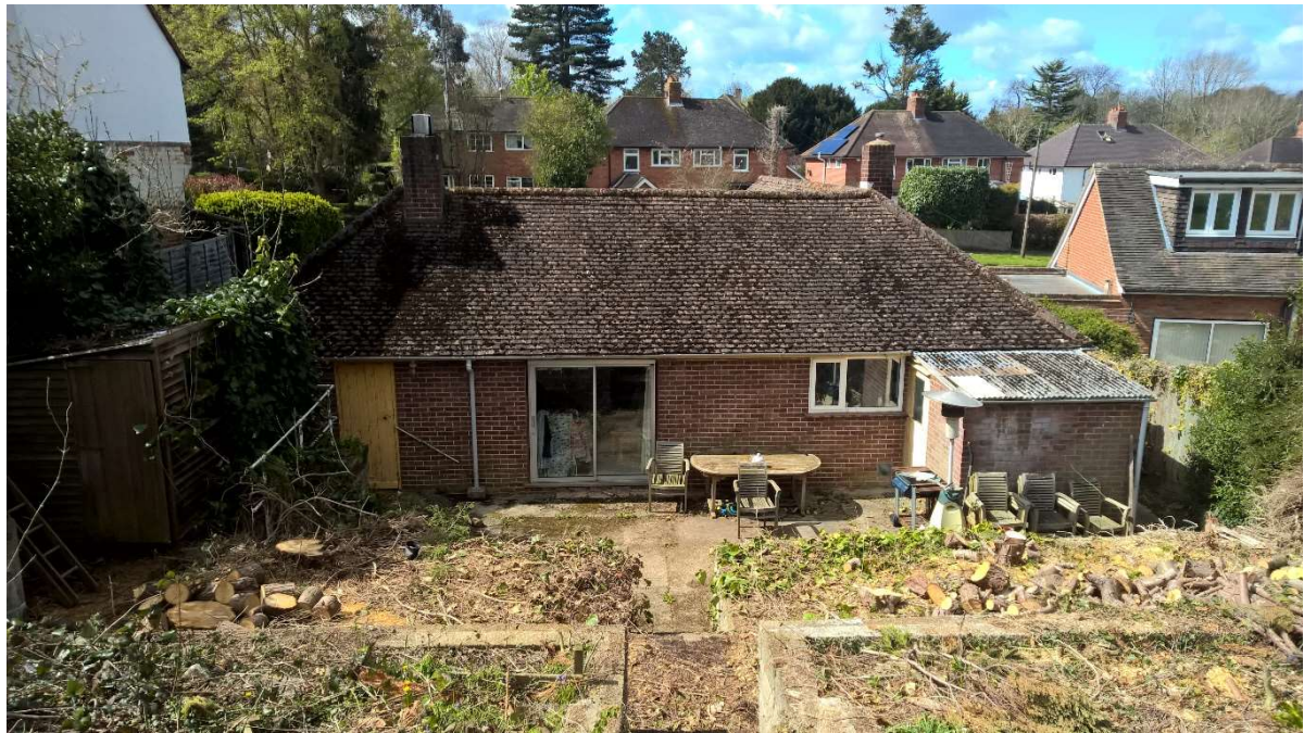
Rear Elevation (above) viewed from tiered garden following the clearance of several Fir Trees.
