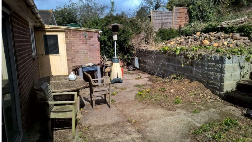
Existing lean-to extension (above).
