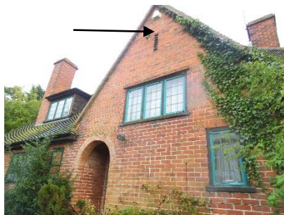
Plate 3.8: Location of a potential roof void
