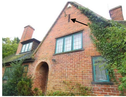
Plate 3.2: Brick gable-end in the northern elevation with potential access point into the building for bats through the vent
