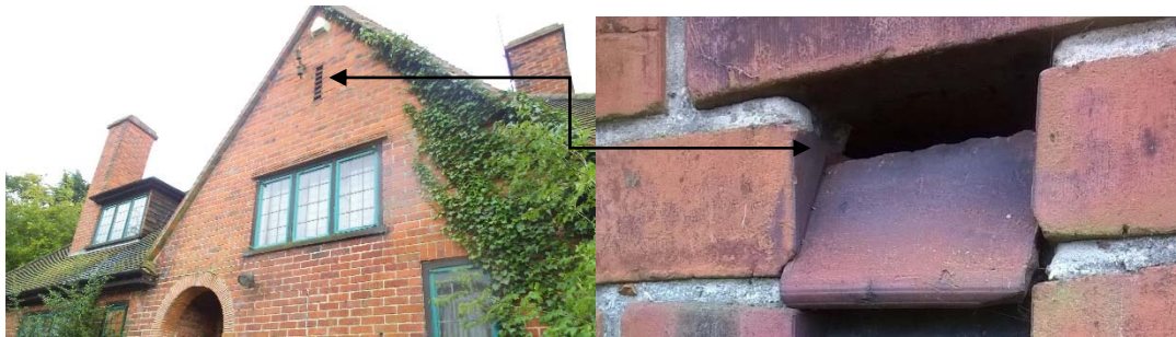
Plate 8: Vent feature providing access into a wall cavity
