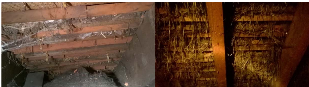
Plate 2: View of the clay roof tiles fitted directly onto the wooden rafters
