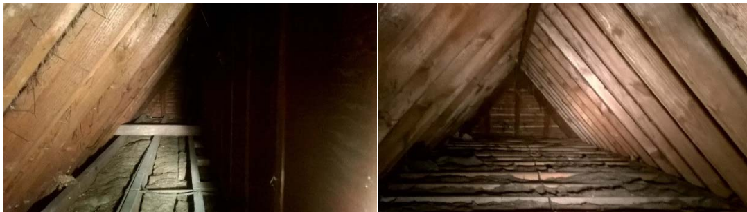
Plate 1: Internal view of the unconverted loft spaces
