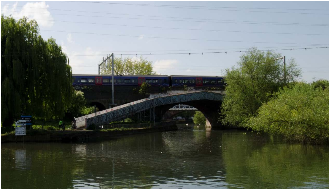
Figure 3.4: Stepped Horseshoe Bridge
