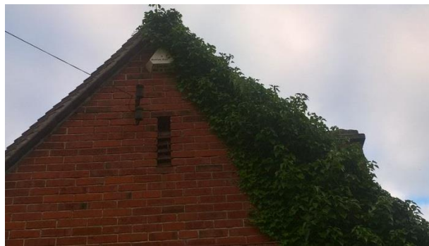
Plate 4.6: Vent Features on Southern Gable End
