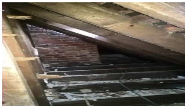
Plate 4.4: Coomb Space Around Perimeter of Roof
