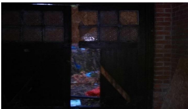
Plate 4.7 Broken Garage Door
