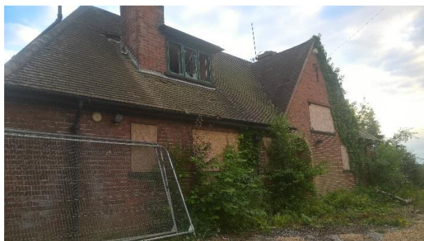
Plate 4.1: Northern Elevation of Main House
