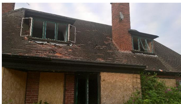
Plate 4.2: Southern Elevation of Main House
