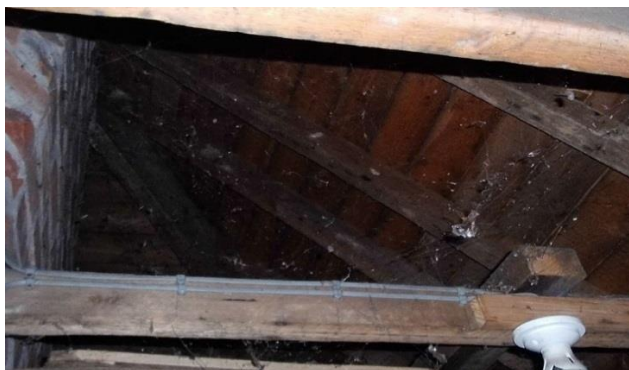
Plate 4.9: Cobwebs and Beams in Roof Void.
