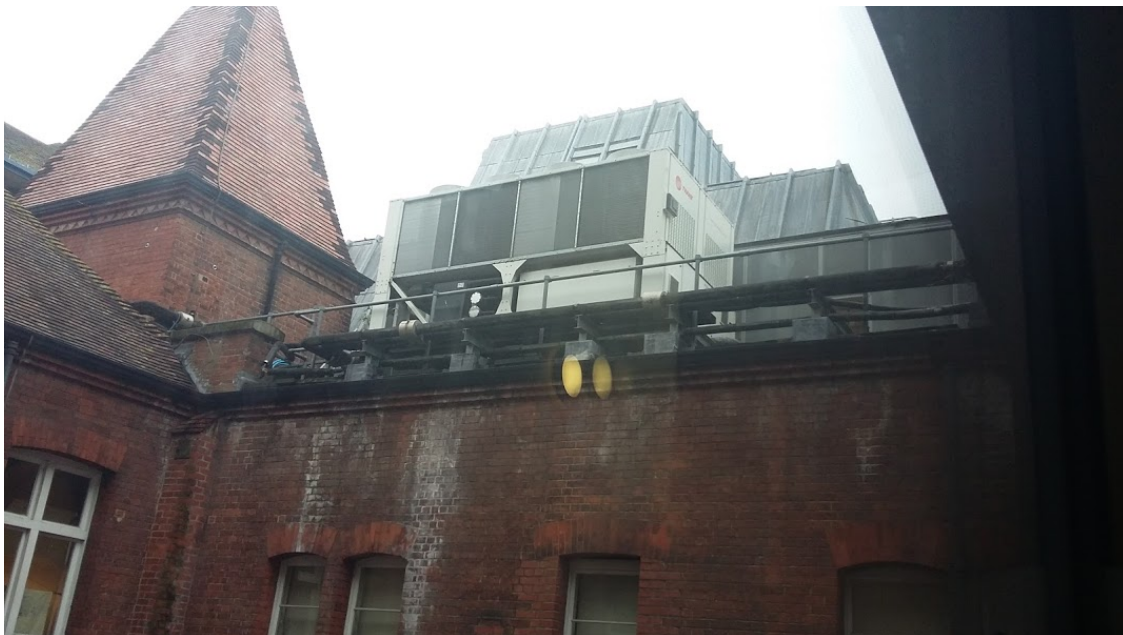
View of the existing Chiller Plant from the courtyard
