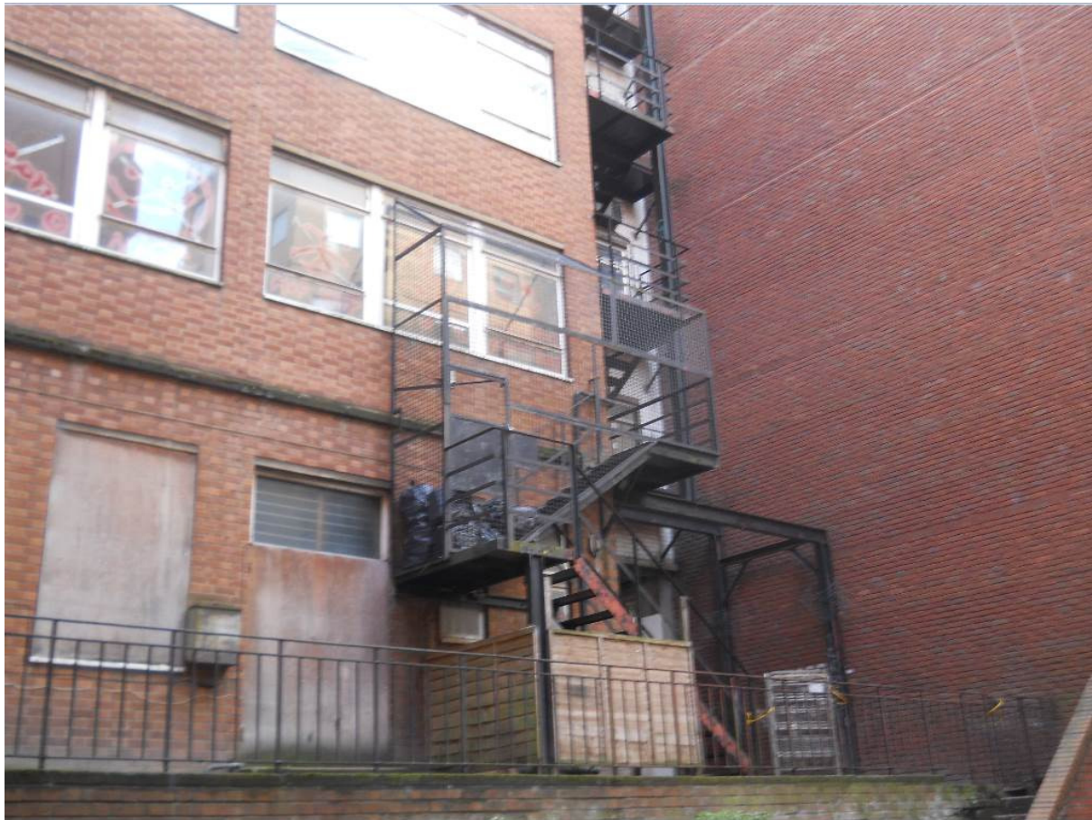
PLATE 3: REAR OF 29-35 STATION ROAD FACING EAST
