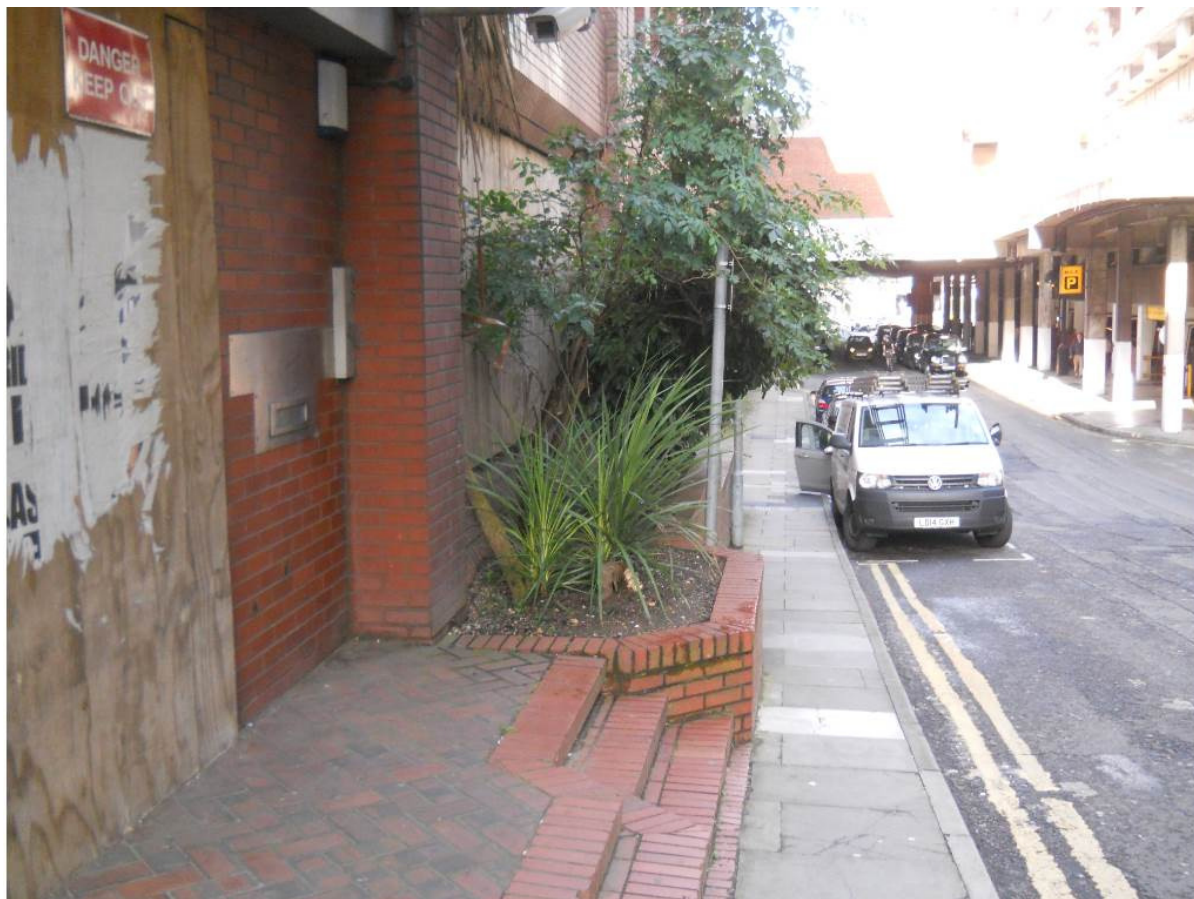
PLATE 6 : ENTRANCE TO GARRARD HOUSE FACING WEST
