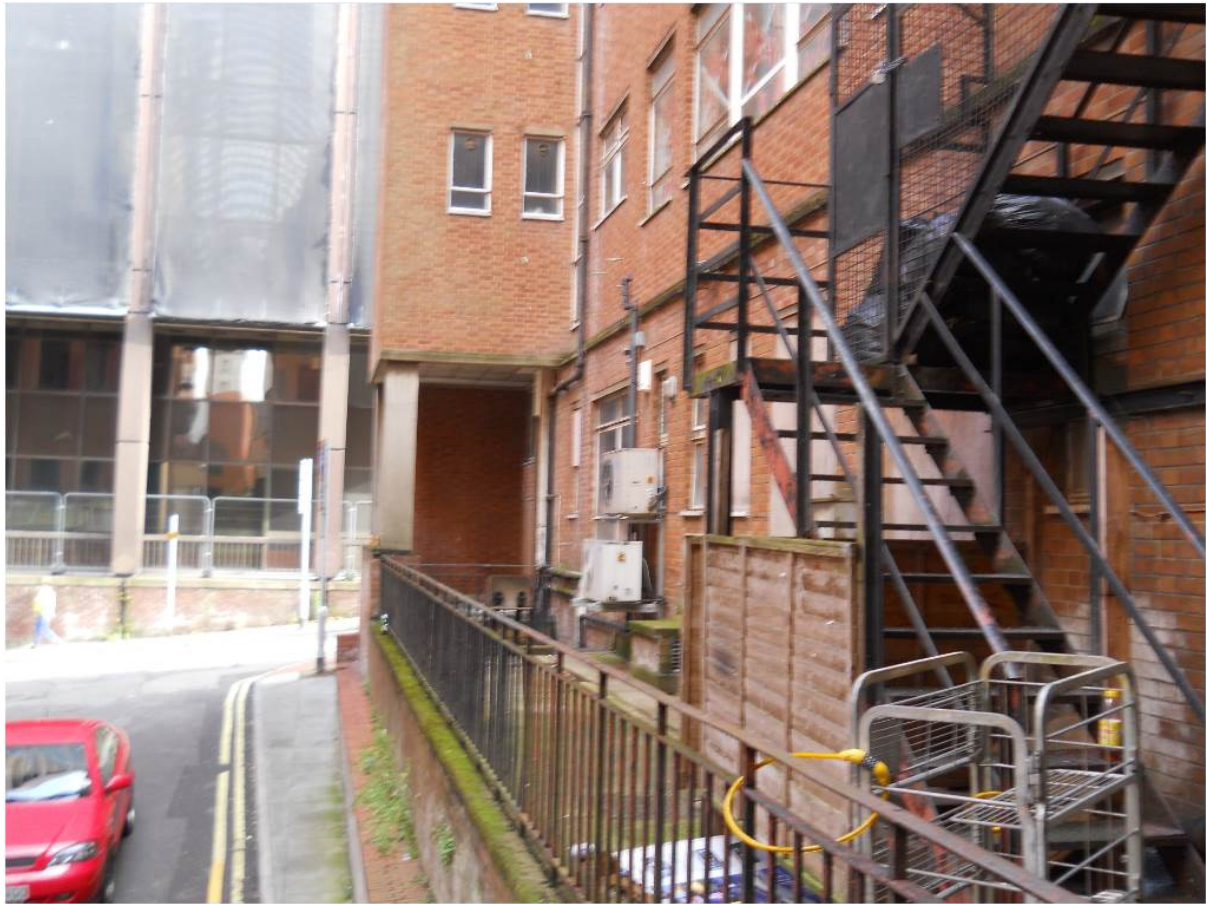
PLATE 2 : REAR OF 29-35 STATION ROAD FACING NORTH
