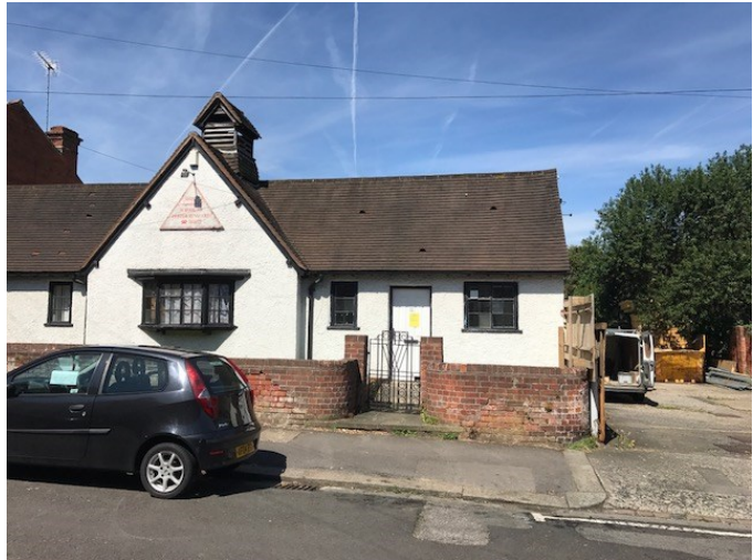
Photo 2 No. 12 Shaftsbury Road
